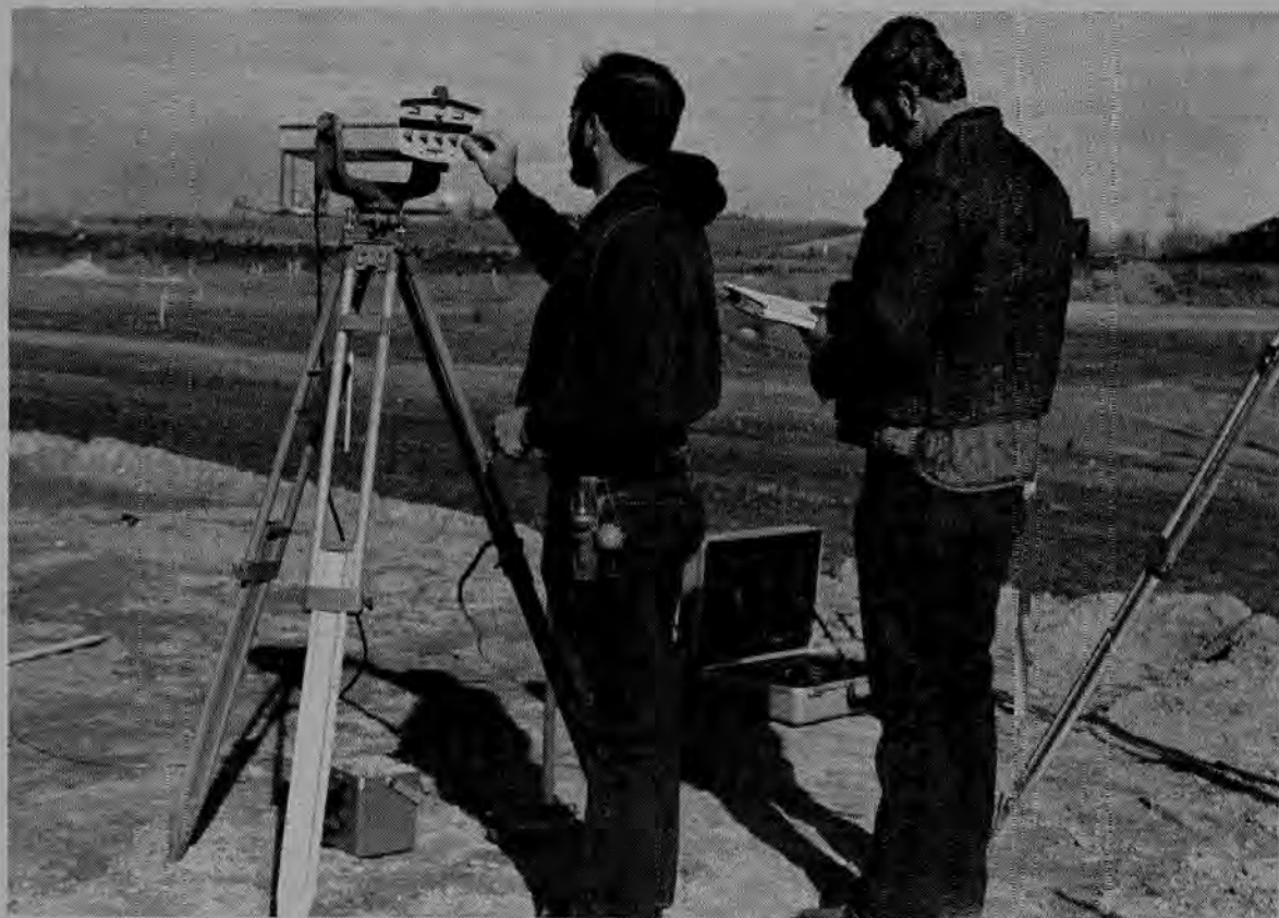
CONSTRUCTION CONTROL Inc. of Marysville at work on the Linda Mall project. Local 3 crew Charles St. Maurice Jr. (right) and Jim Miller (left) are using the latest equipment in measuring distance. The model 3800A is a direct read out instrument with a range of 10,000 feet. Visual display of the total measured distance in feet, corrected for atmospheric conditions, is accomplished in less than
