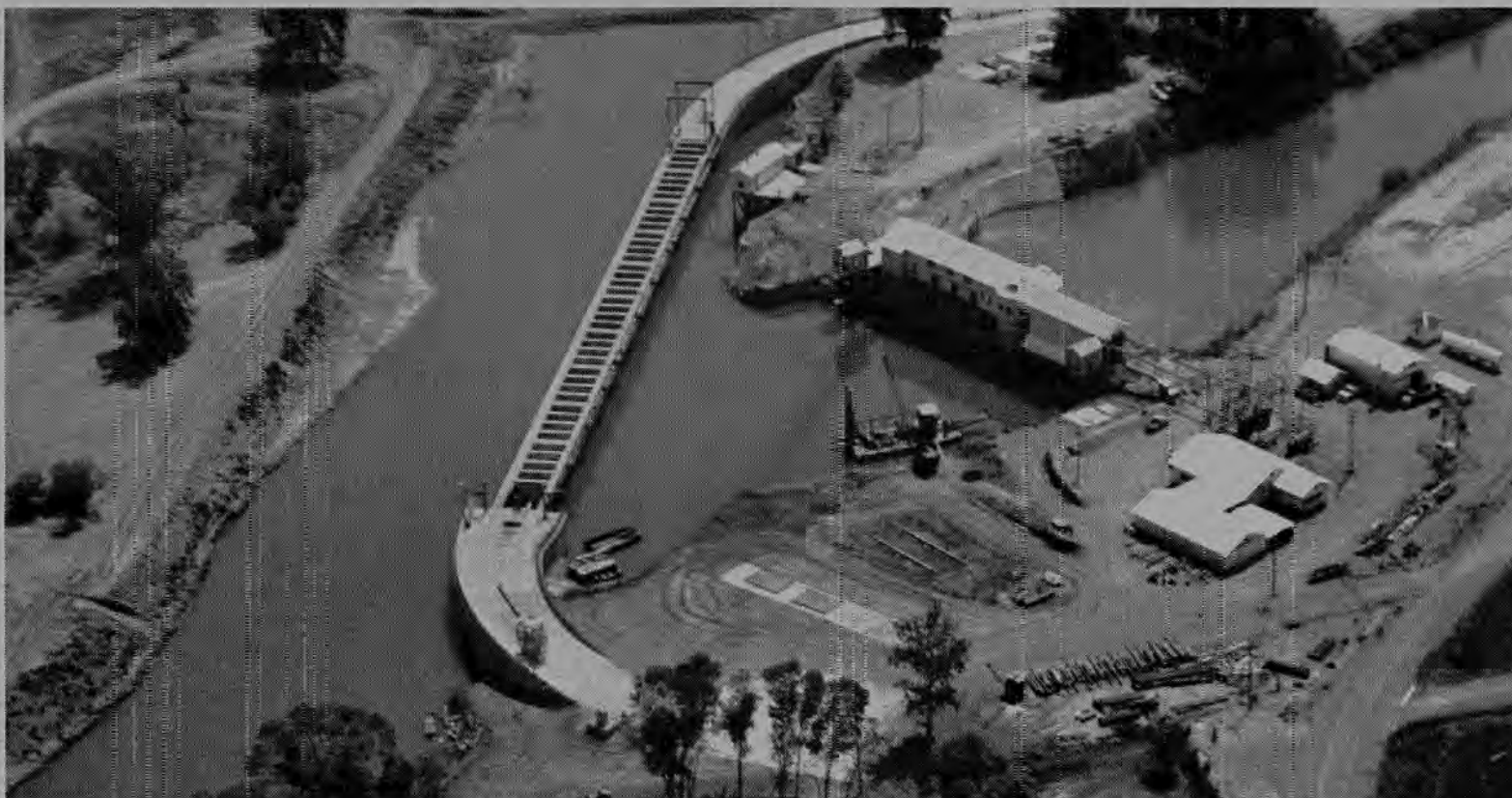
AN AERIAL VIEW of the new Glenn-Colusa Fish Screen shows the pumping plant (right) spanning the canal, the mammoth 25,000 pound capacity traveling hoist used to move screens (top) and a
