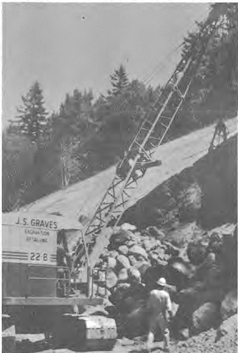
A $250,000.00 EXTRA work order was needed to repair rain damage on Darkenwald Construction Company's Pt. Reyes road spread. Several of the big cuts slipped and covered the roadbed and had to be mucked out and rip-rap moved into the slopes. Shown above moving rock is John Graves, operating, and Warren Harrelson, oiler.
