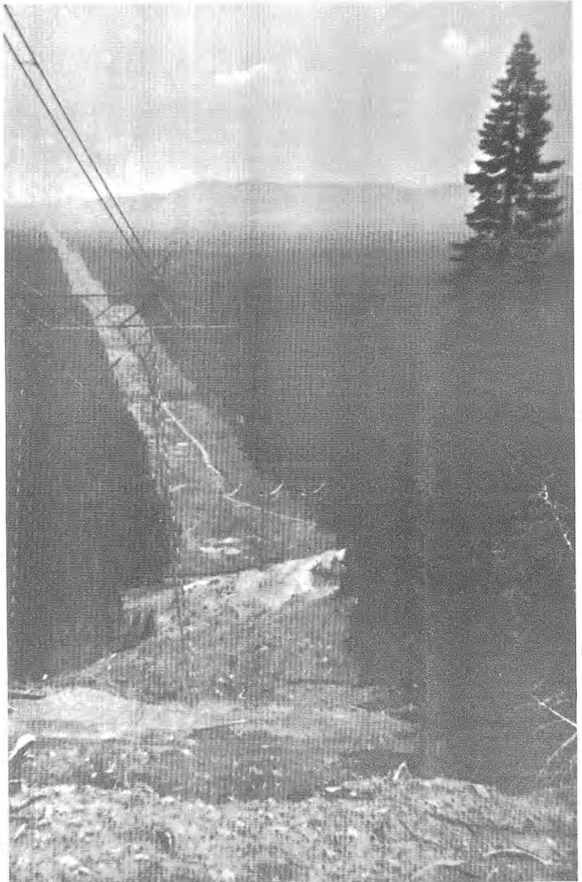
BUREAU OF RECLAMATION transmission line running from the Oregon line to Round Mountain, approximately 90 miles over rough and rugged terrain. Power City Construction Company.
