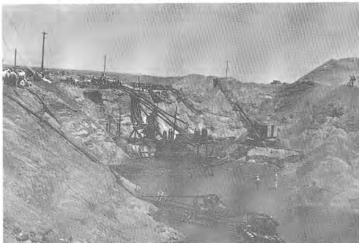
NORTH PLATTE RIVER gets a face-lifting from a Bucyrus 30B model during the digging of the sump for spillway of the Kingsley Dam near Agalala, Nebraska in 1937. Operator was Troy Manzer, a long time member of the Operating Engineers, who now resides at 1613 Merian Drive, Pleasant Hills, California. Brother Manzer sent the
