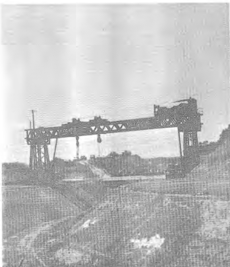
THE BIGGE GANTRY above is also being used by Fredrickson Watson Construction Company on the Corning Canal to raise and lower trimmer and slip form paver over the structures that have been erected.
