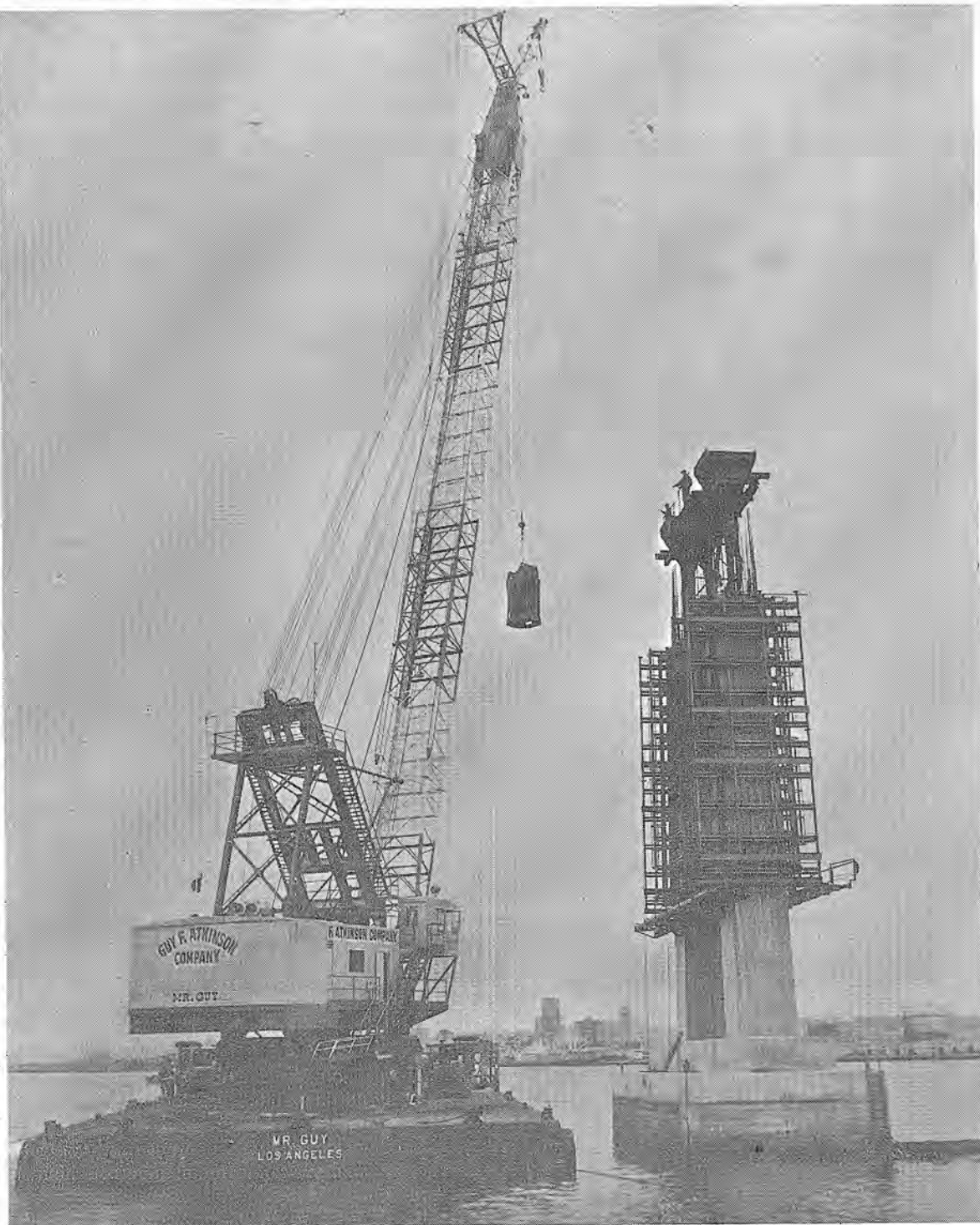
MEET "MISTER GUY" the million dollar derrick built by the Guy F. Atkinson Company and now at work on the construction of the Humboldt Bay Bridge between Eureka and Samoa. The powerful
