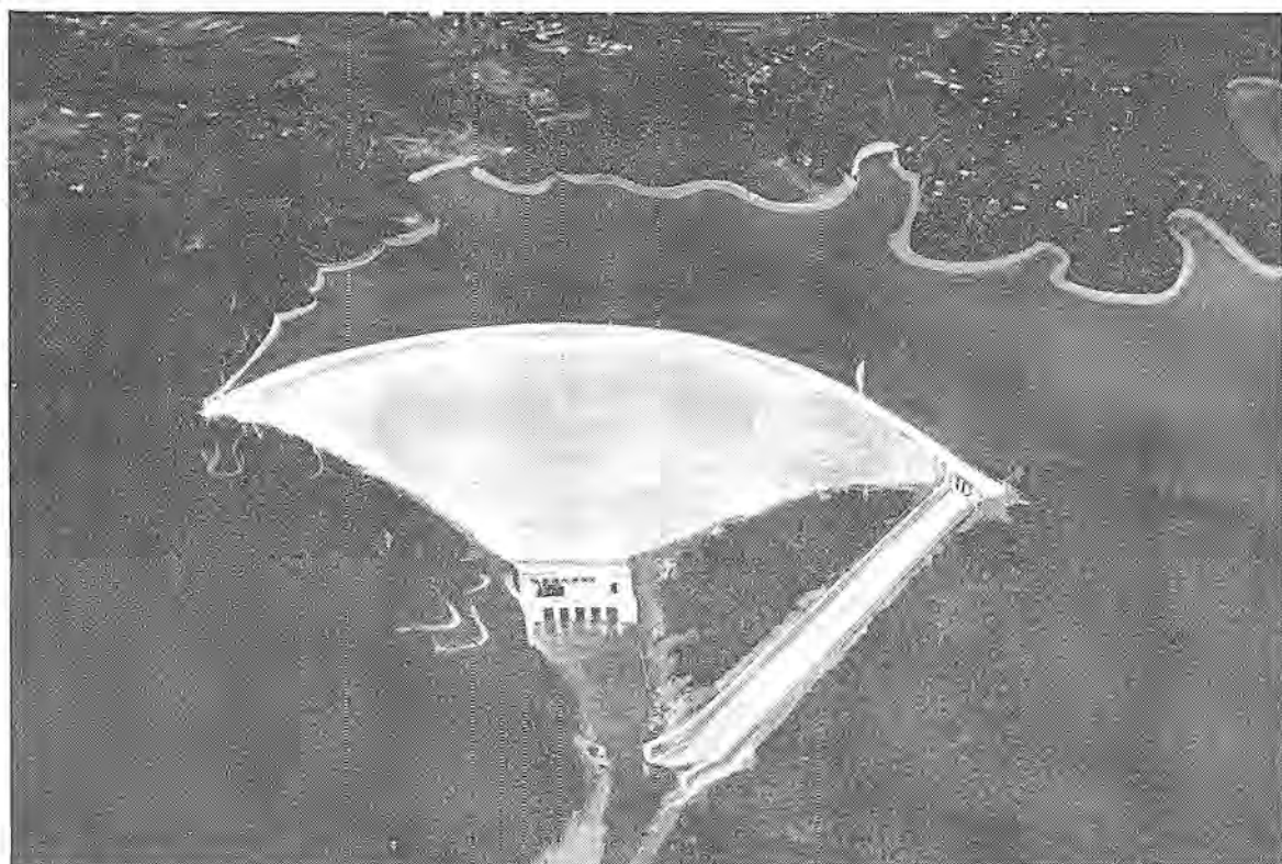
The new Auburn Dam to be constructed on the north fork of the American River will be a thin-arch concrete structure, as shown in this artist's concept. It will be the fourth highest in the U.S.
