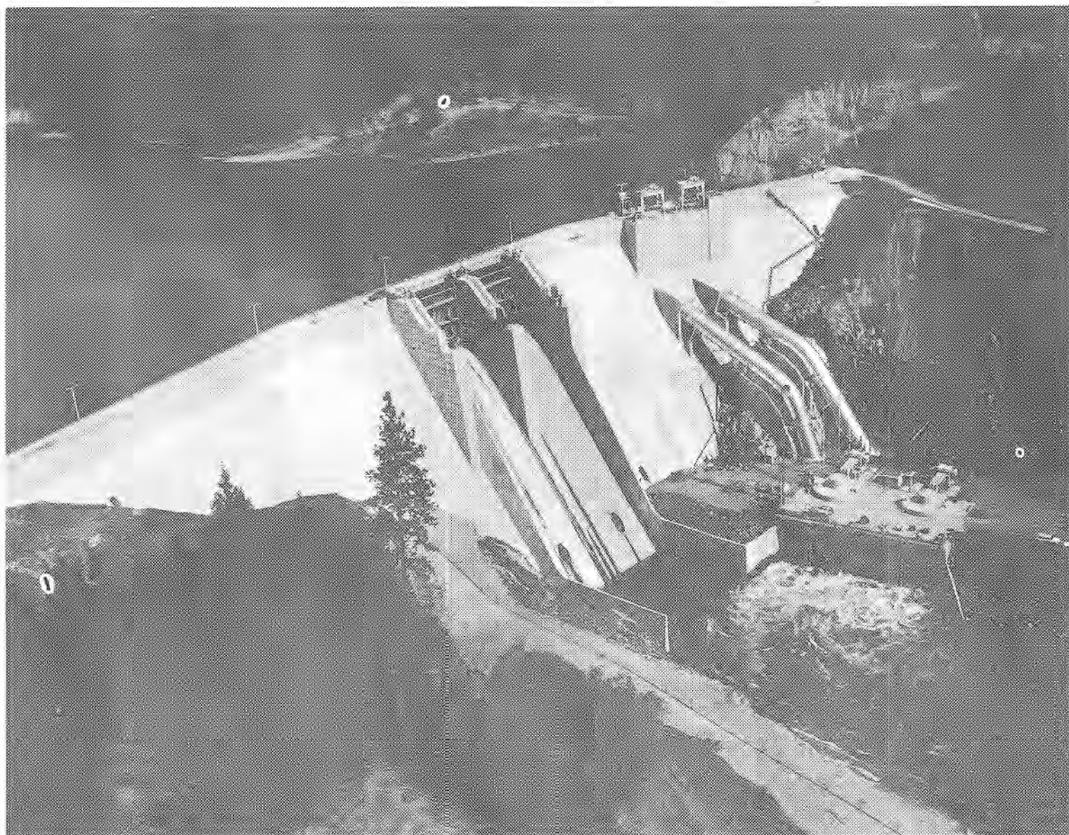
PG and E's new dam, rising 248 feet from bedrock, has crest length of 907 feet. It contains nearly 251,000 cubic yards of concrete. Plant generates 101,000 kilowatts for public, industry.
