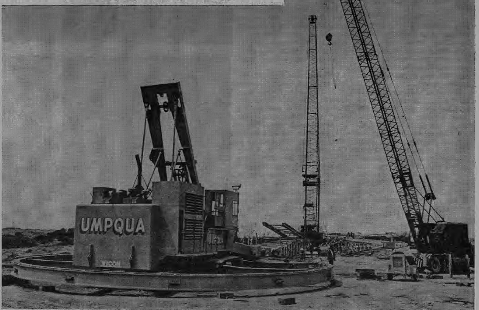
MANITOWOC 4600 RINGER being assembled on Humboldt Bay South Pit.
