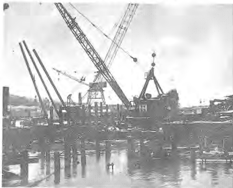
The old pilings come out and new "H" beam pilings go in as Healy-Tibbits constructs pier for Bethlehem Ship Yards, San Francisco.
