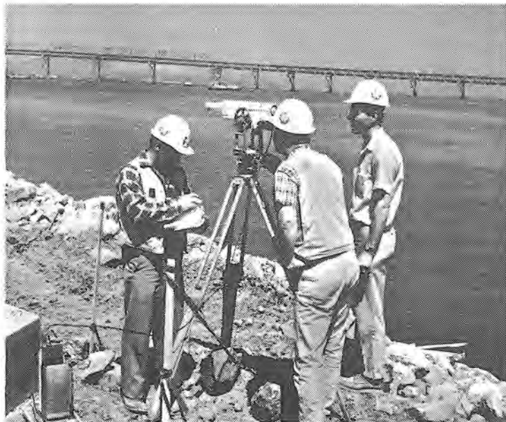
Dimitri Keriotis, party chief; Jerry Clow and Eugene Schaufler, set up laser beam for aligning the huge BART trans-bay trench.
