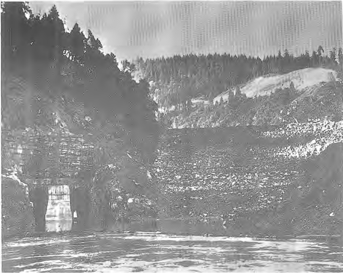
Perini Yuba Associates have completed the diversion tunnels and coffer dam preliminary to the start of construction on Bullard's Bar Dam, which will add to the state's over-all flood control plan.
