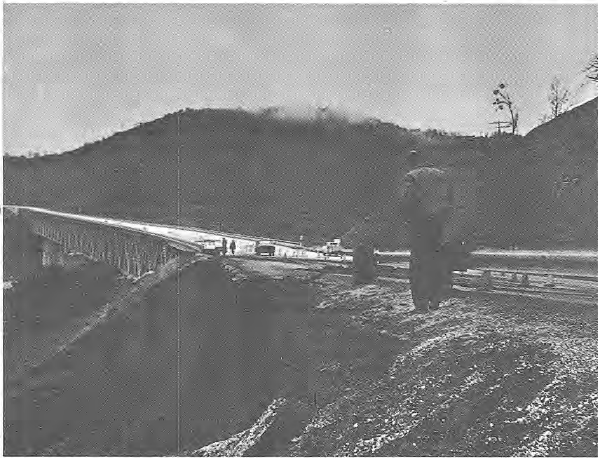
EARTH SLIDE This is a view of the highway 70 slide on the upper end of the West Branch bridge where a 150 foot strip of pavement was undermined and slipped into Lake Oroville. Division of highways engineers stated the slide has forced
