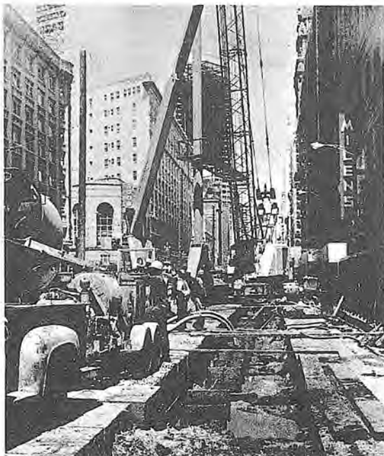
Constructing "slurry wall."
