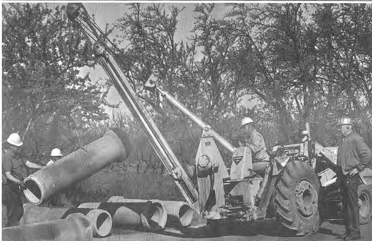
WATCHING HIS BRAINCHILD at work is Brother Gene Favretto, an Operating Engineer, Local Union No. 3, for 27 years, an inventor of the Marvin Tac/Boom attachment for the standard Backhoe. Brother Paul Hawkins of Santa Rosa is the operator on the Kirkwood, Bly and Wood pipe job at Lodi, California. Brother Hawkins is
