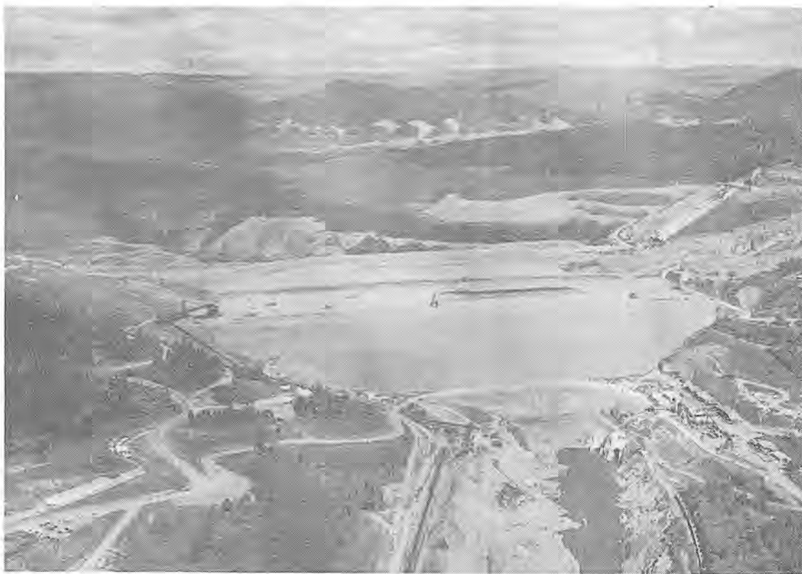
OROVILLE DAM —Shown here is 40 million cubic yards of earth-fill marking one-half of completion of world's largest dam of this type. Picture shows McNamara-Fuller powerhouse at right; Langenfelder clearing in background; reclaim tunnel, conveyor system and spillway also shown.
