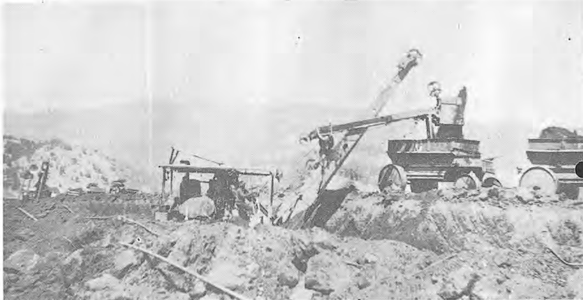
DAM SITE —this looks like tandem the wagons backed up to a Northwest shovel. Master Mechanic was Harry Eck and shovel runner was Brother Bill Raling. The project looks like part of Gordon Valley Dam, about '24 or '25.
