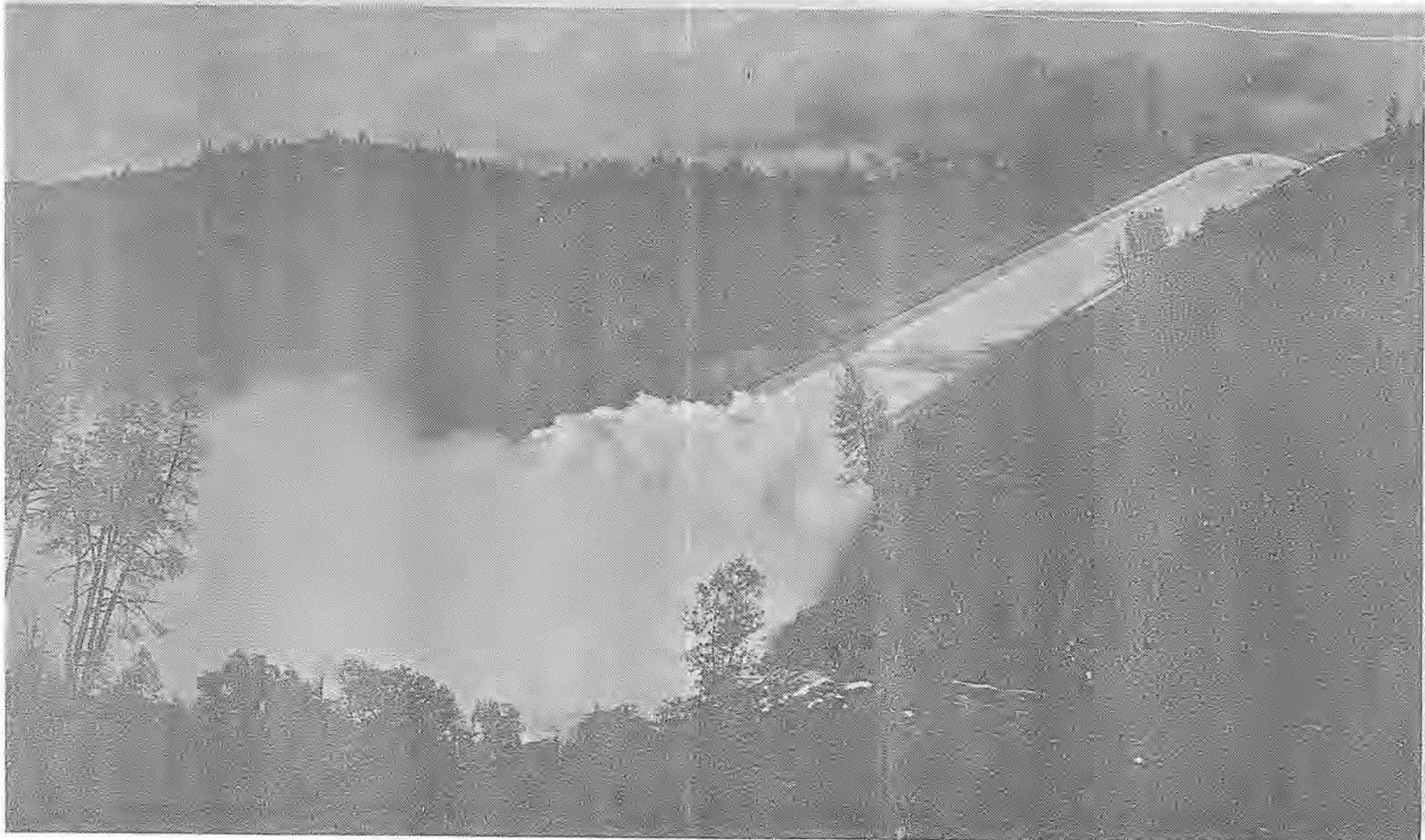
SPRAY SPECTACULAR as water bursts out the spillway at Oroville Dam at a speed comparable to 37 miles per hour as it is released from the reservoir behind the huge dam. The spray and turbulence at left is caused by concrete teeth called "energy dissipaters," which break the force of the spillway water, sometimes shooting it as high as 200 feet. The level of Oroville Lake was 850.86 feet
