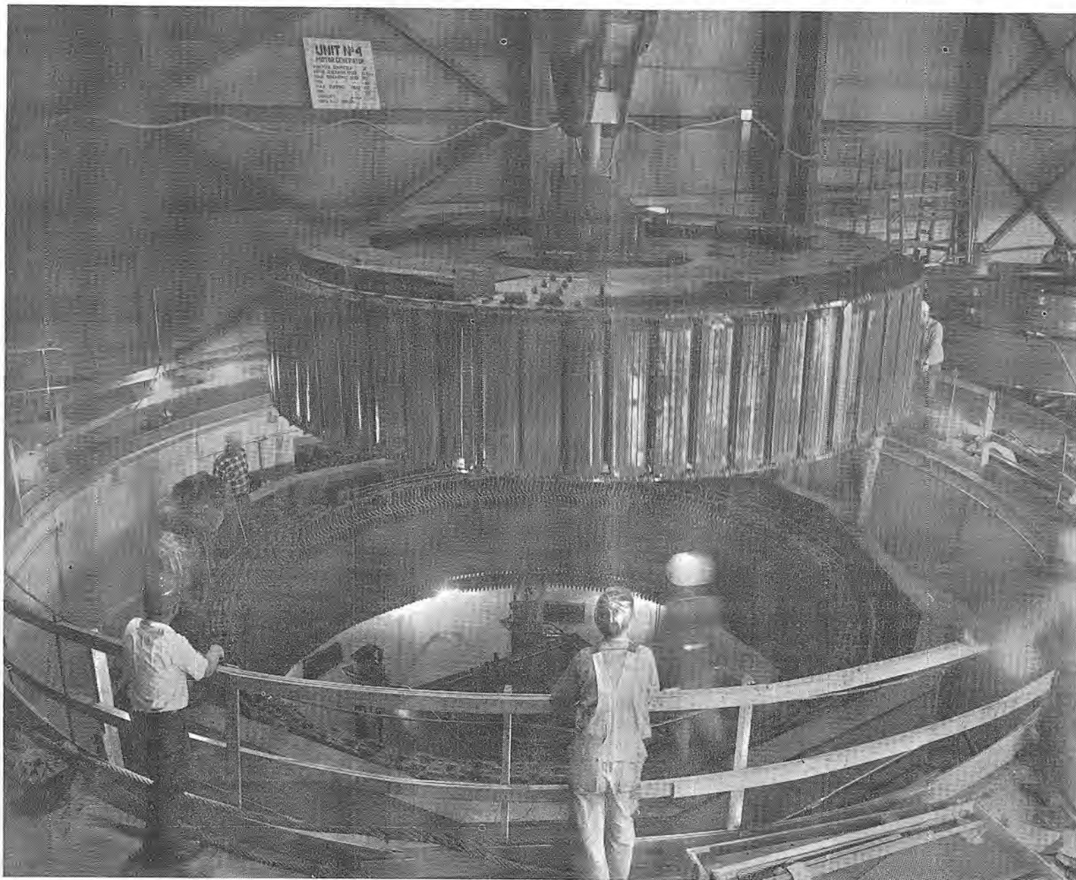
HUGE ALLIS CHALMERS Synchronomus motor hydro generator rotor being placed into position with 150-ton American overhead crane. Overall diameter of motors are 36 feet developing 40,000
