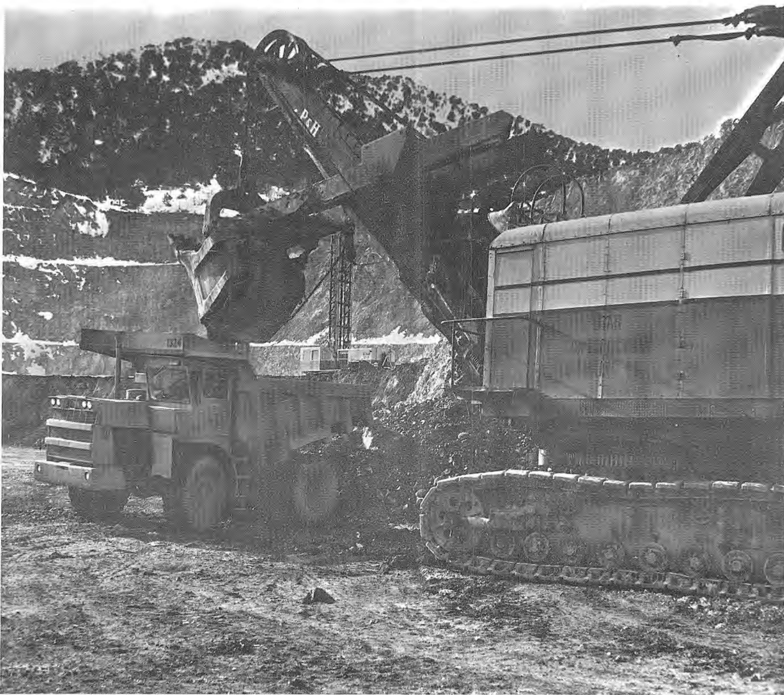
UTAH CONSTRUCTION & Mining Co., Cedar City Operations. Waste removal at our Comstock Mine with a shovel having a bucket capacity of 6 cubic yards of waste, loading into a 32-ton truck
