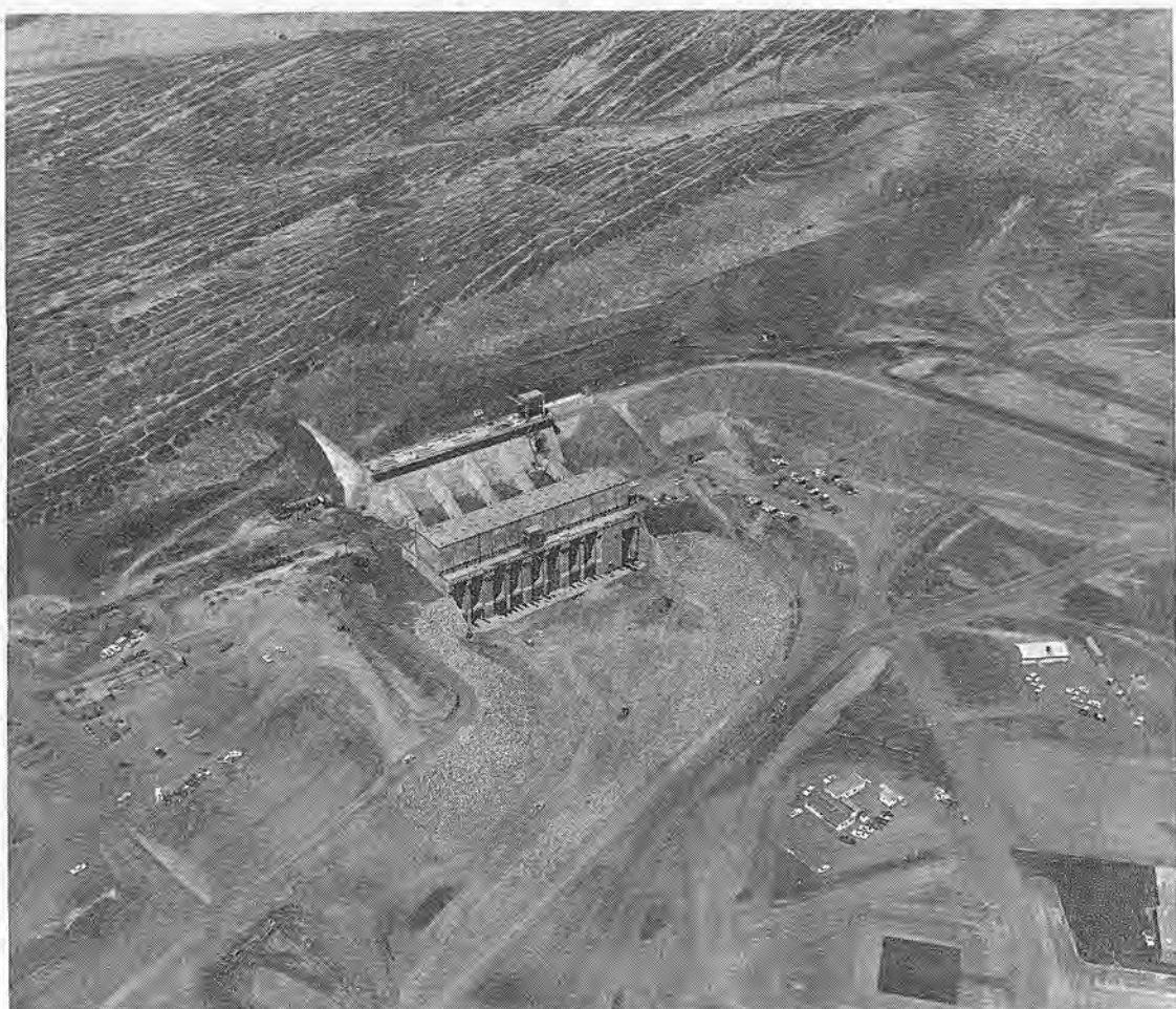
COMPLETED THERMALITO powerhouse taken early in September 1967. Overhead cranes on intake and exhaust sections of system are used for raising and lowering of debris gates to keep obstacles out of turbines. Rip-rap was completed
