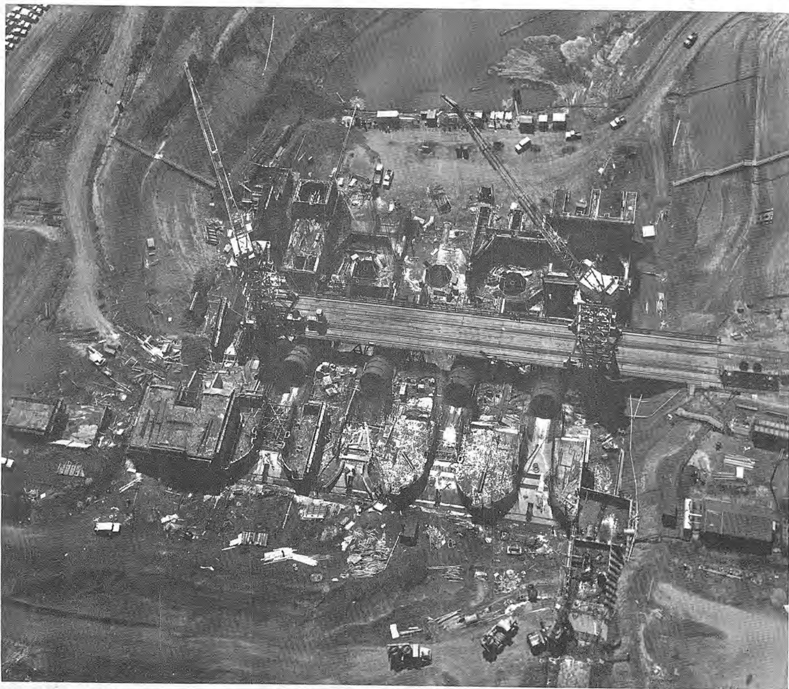
THERMALITO START shows operation of two 50-ton Clyde Whirly Cranes in photo being shown pouring concrete at Thermalito
