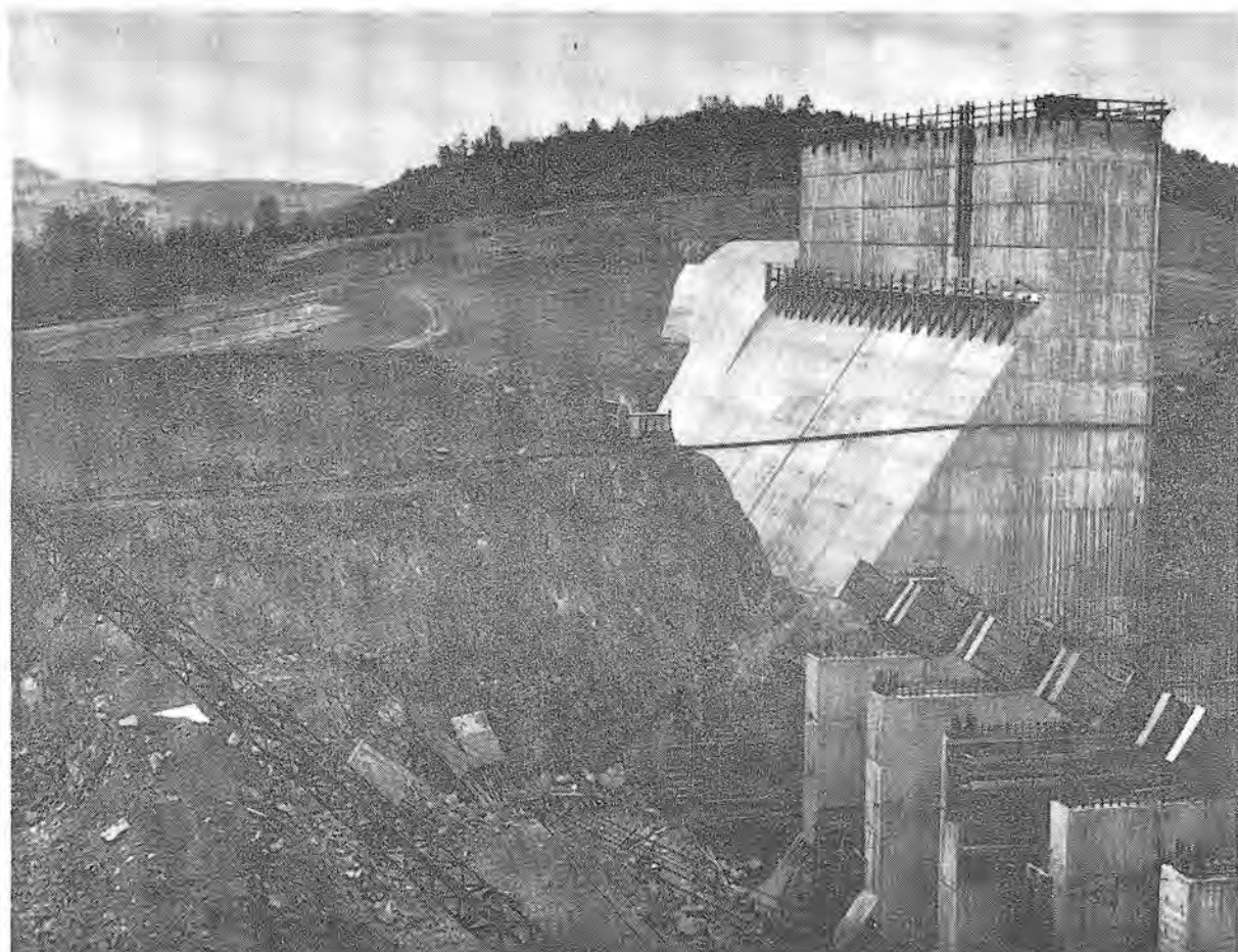
Spillway gates and emergency overflow are nearing completion at Oroville Dam. Riprap from the spill-
