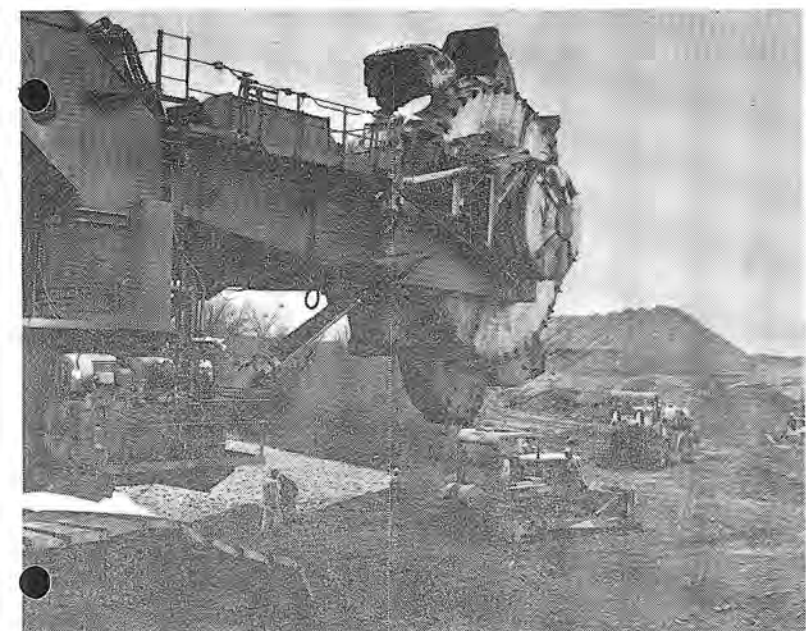
"The Wheel" moves slowly across the Feather River to begin another assault on the cobble pile. The Wheel loads 6,000 tons an hour.
