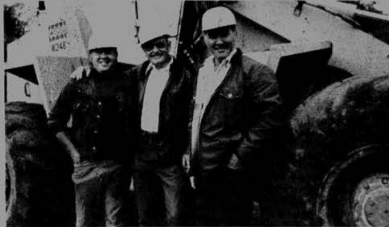
THE CENTRAL VALLEY SEWER project in District 70 continues, as the new trunk sewer mains are being laid. Shown above are Ed Benz, job steward for Glen Shook, Inc., owner Glen Shook and Superintendent Bud Cox.
