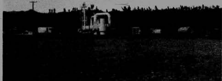
A NEW ROCK SAND and gravel operation, owned and operated by W. Jaxon Baker, recently received a use permit with the help of brother engineers in the Redding area. Shown above is the new hot plant.
