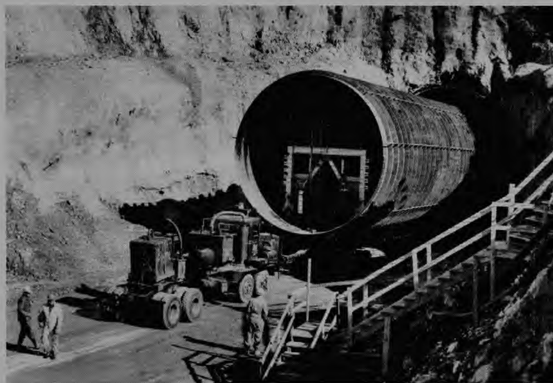
EIGHT INCH CLEARANCE with a 12 degree grade this 80 foot long, 23 ft. diameter steel liner at New Melones main diversion tunnel. was a task solved by Bigge Drayage to position
