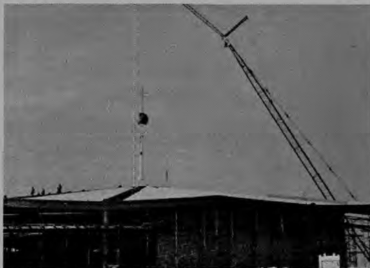
ON TOP OF THE WORLD —A new 59-foot steeple has been installed by San Jose Crane and Rigging atop San Jose First Baptist Church's $2½ million Sanctuary. It is being built by Oscar W. Meyer on the site of the old Ironwood Golf Course. The steeple, rising 119 feet above the ground, dominates the 35 acre site on a hillside. Steel substructure of the steeple is surmounted by a large globe on which rests a large cross. Operator for the placement of the steeple was Fred Hoerman working with oiler Donald Freitas. The main building includes a 2,200-seat auditorium, offices, chapel, library, nursery, kitchen, and will replace the original downtown church which was constructed in 1850. Present congregation numbers 3,800 to use facilities of the new four-story church.
