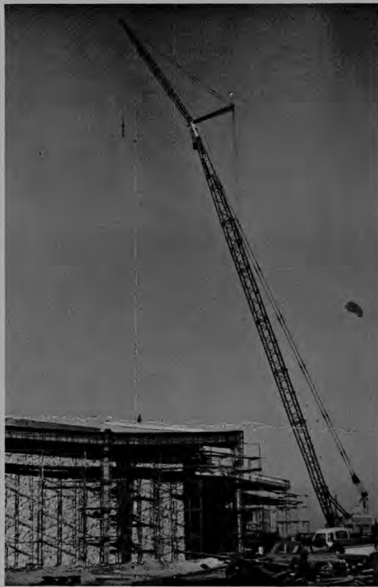
ON TOP OF THE WORLD —A new 59-foot steeple has been installed by San Jose Crane and Rigging atop San Jose First Baptist Church's $2½ million Sanctuary. It is being built by Oscar W. Meyer on the site of the old Ironwood Golf Course. The steeple, rising 119 feet above the ground, dominates the 35 acre site on a hillside. Steel substructure of the steeple is surmounted by a large globe on which rests a large cross. Operator for the placement of the steeple was Fred Hoerman working with oiler Donald Freitas. The main building includes a 2,200-seat auditorium, offices, chapel, library, nursery, kitchen, and will replace the original downtown church which was constructed in 1850. Present congregation numbers 3,800 to use facilities of the new four-story church.
