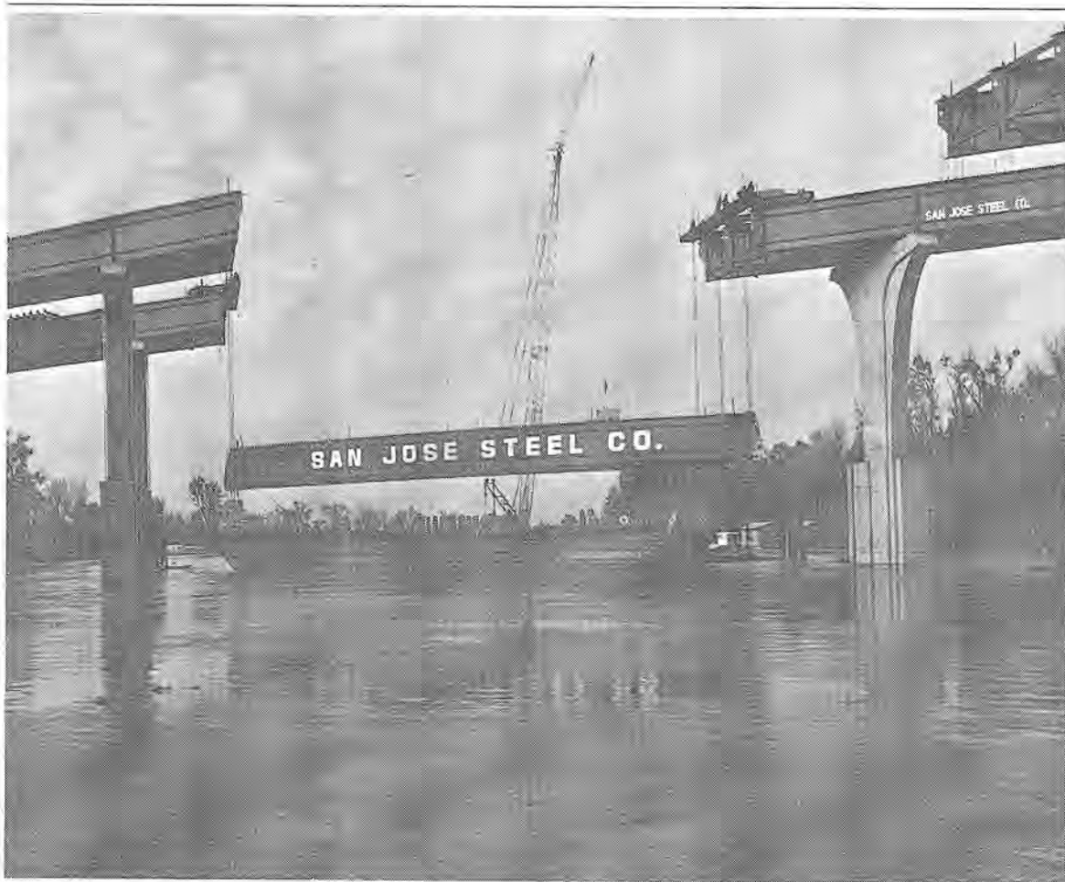
BRIDGING the Sacramento River at Elkhorn Ferry called for a unique technique as the San Jose Steel Company lifted the final beams into
