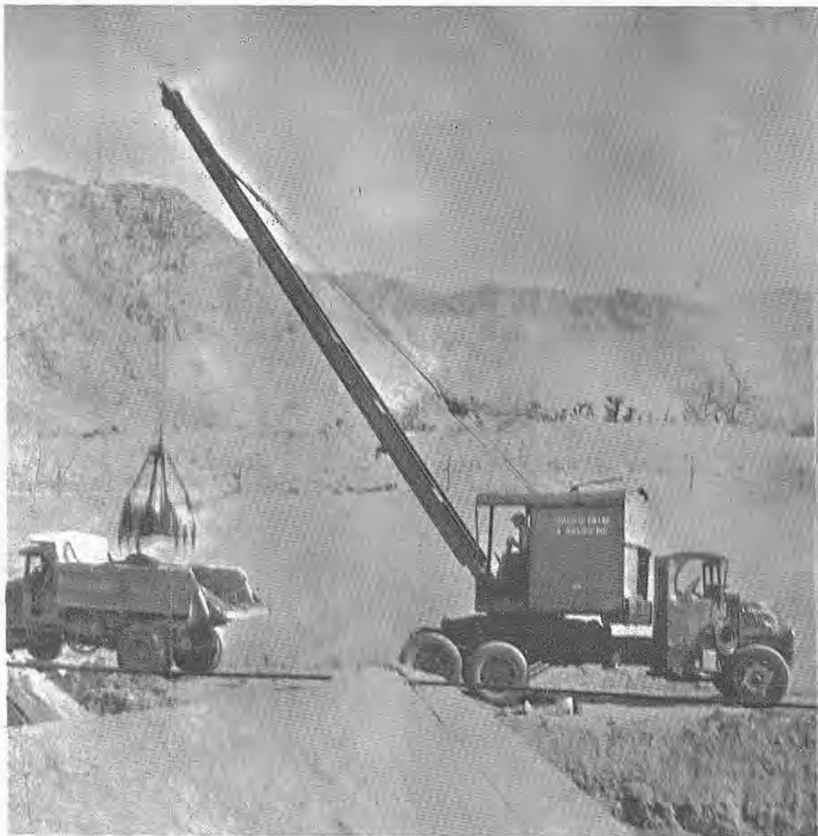
PACIFIC CRANE & RIGGING married a Universal to a 1919 Mack Truck to produce this unique outrigger shown at work on the Los Angeles Aqueduct in 1937. Outriggers were unheard of at the time and this one boasted a 40-foot steel
