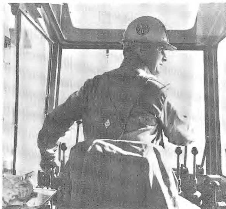
Rex Richardson skillfully operates levers in control cab as the orange peel picks up huge rock. Rocks are placed one at a time.
