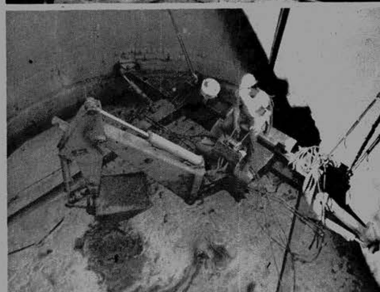
TWO-PART BACKHOE is run by Pat DeRego in the above photo. The mounting of the backhoe unit of the John Deere 500-C (top photo) inside the 22-foot-diameter substation was necessitated by large amounts of rock which could not be removed with a clam.
