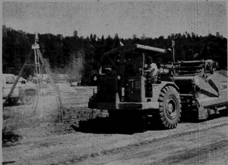
SPACE AGE TECHNOLOGY —Lee Haven, owner-operator, is seen above in the seat of his laser-controlled 613 Cat scraper now at work in the Redding area.
