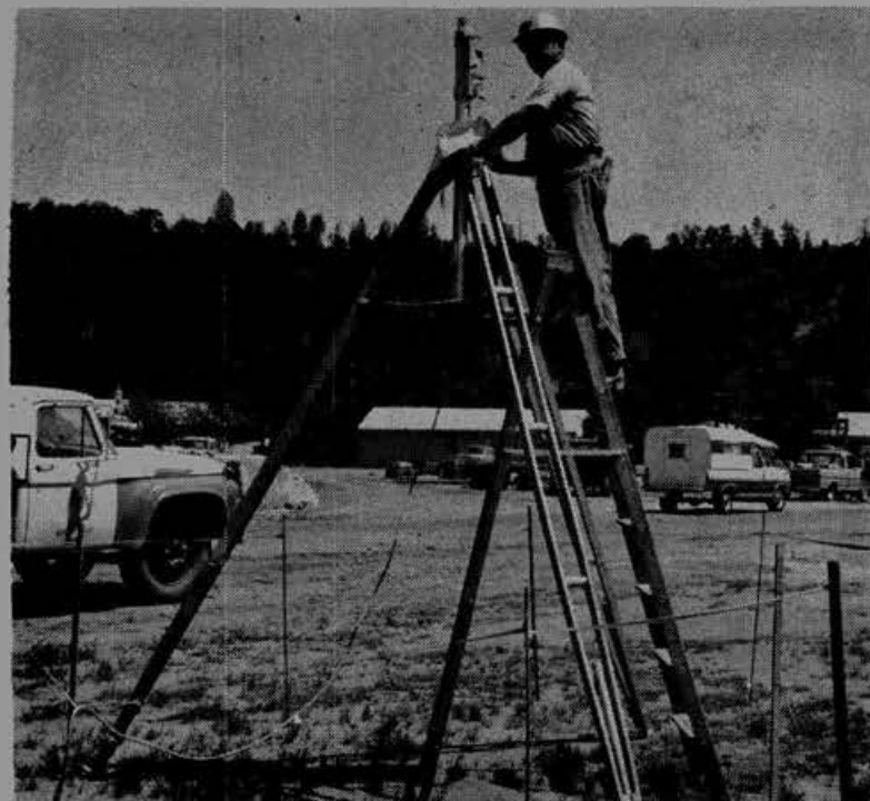
LASER COMMAND POST for Lee Haven's Cat 613 scraper is set up by gradesetter Joe Craig in preparation for work on the Crystal Lake Fish Hatchery.
