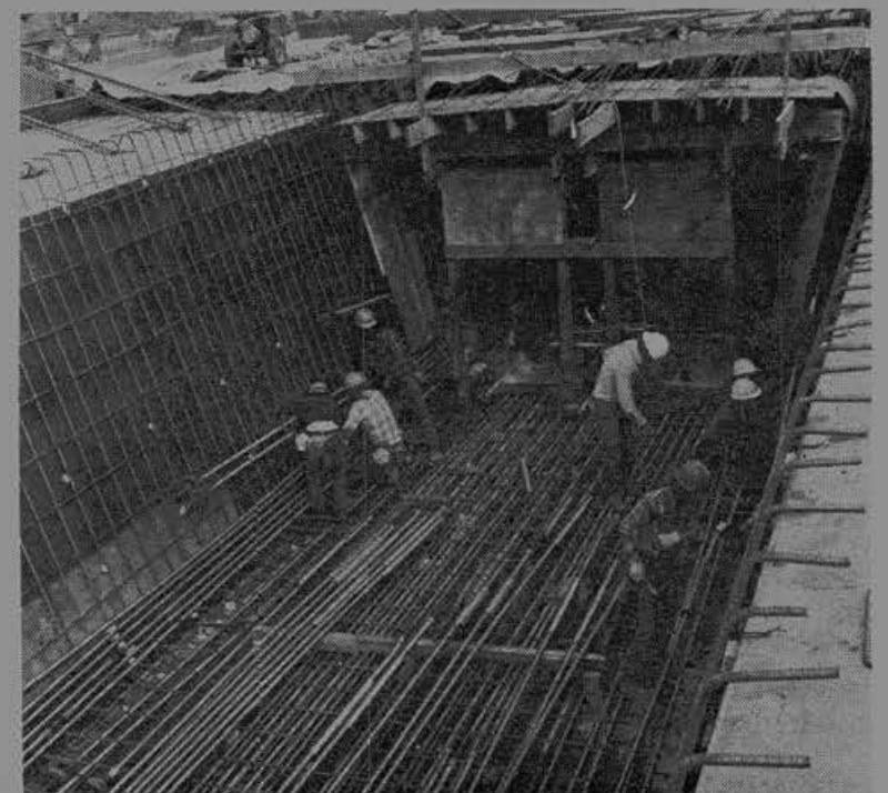
CONSTRUCTION of the new Eel River Bridge is seen in the top photo, taken from the existing bridge. The bottom photo gives a close-up of the special German-patent rebar being used in the construction.
