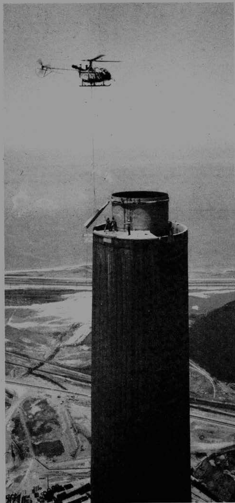
Pictured (attached) is the 1,200 ft. stack at Kennecott Copper Corporation's new smelter. M. W. Kellogg Co. constructed it and is putting on the final touches. The total cost to the new smelter is approximately $280 Million and the stack represents 5 percent of the cost. The Emission Control system goes into operation in 1977. Presently there are approximately 1,150 employees including all crafts, 123 are Operating Engineers. Completion of the project is expected in July 1977 with 42 percent of the project complete at a cost of $122 Million. Kennecott Copper is using single absorption acid plants because they require less maintenance down time and thus achieve greater long-run sulfur capture and better pollution control. EPA regulations developed to insure meeting the ambient air quality standards require compliance by July 1977. The Utah Air Conservation Committee (UACC) variance under which Kennecott Copper is operating expires in July 1977.
