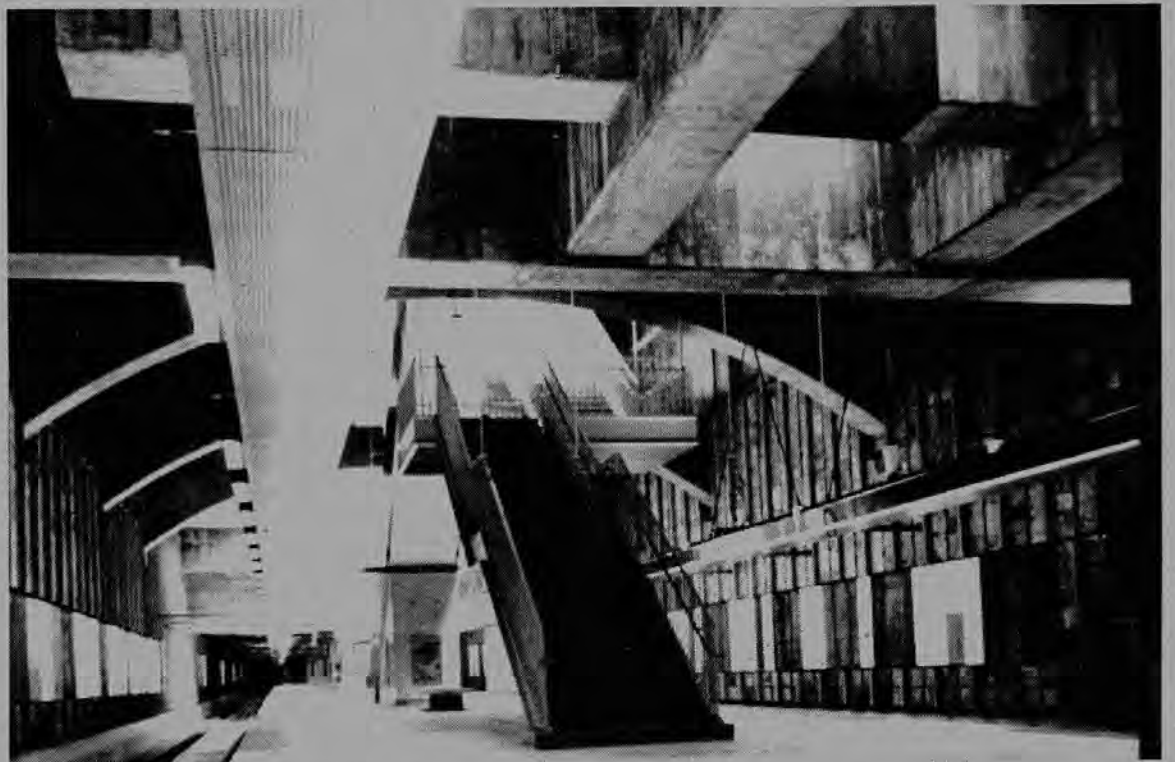
THE GLEN PARK STATION pictured here is a medium size suburban station, consisting of marble walls with translucent interlock-
