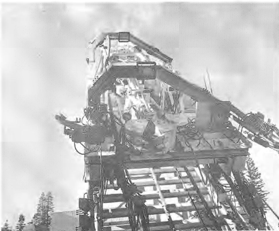
SHOWN ABOVE are pictures of the shaft equipment at the Loon Lake shaft job. This outfit is averaging 50 to 60 feet per week. This equipment also has a Criderman
