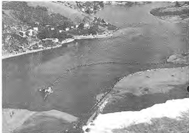
Utah Construction has a 12-inch suction dredge working at Jenner on the Russian River trying to keep the channel open for barges.
