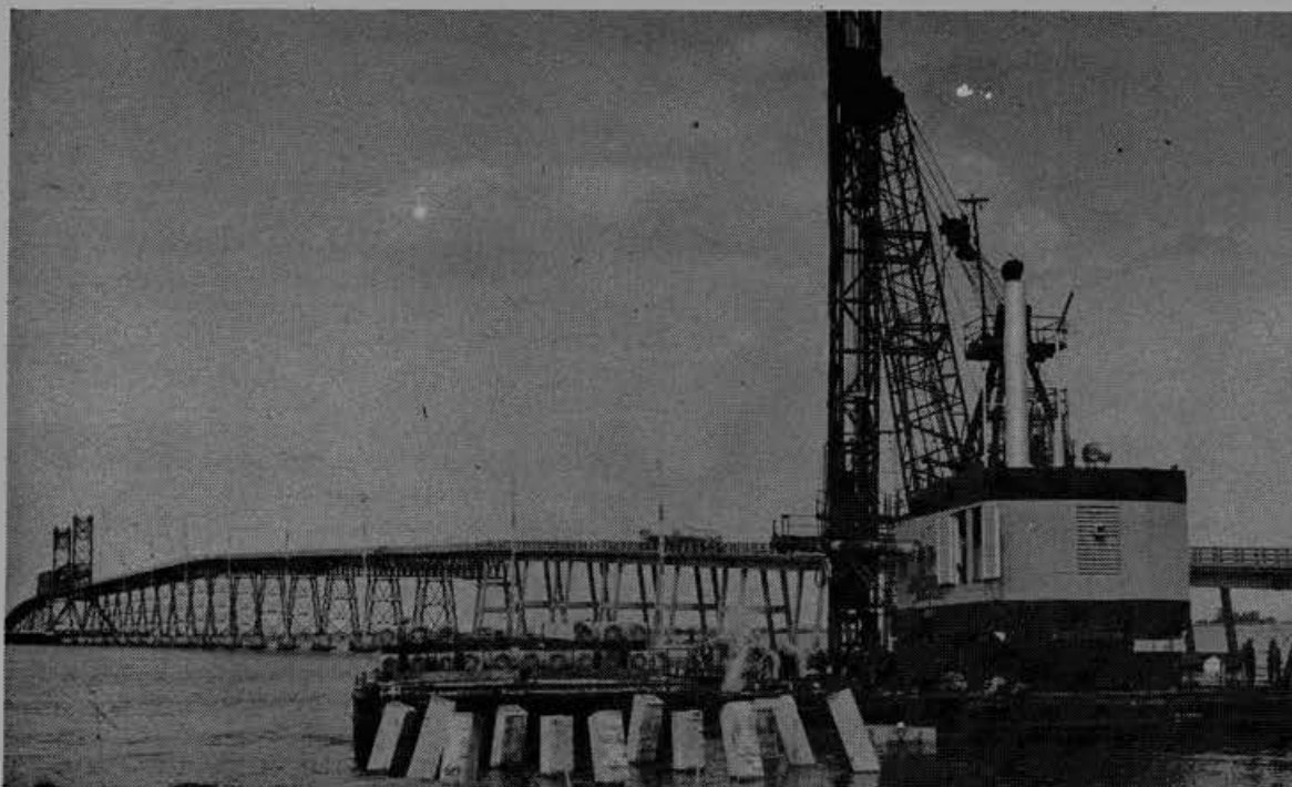
A SEPARATE JOB on Highway 4—the new Antioch Bridge—is now in its early stages and operating engineers operate the cranes for the pile drivers. The big floating crane
