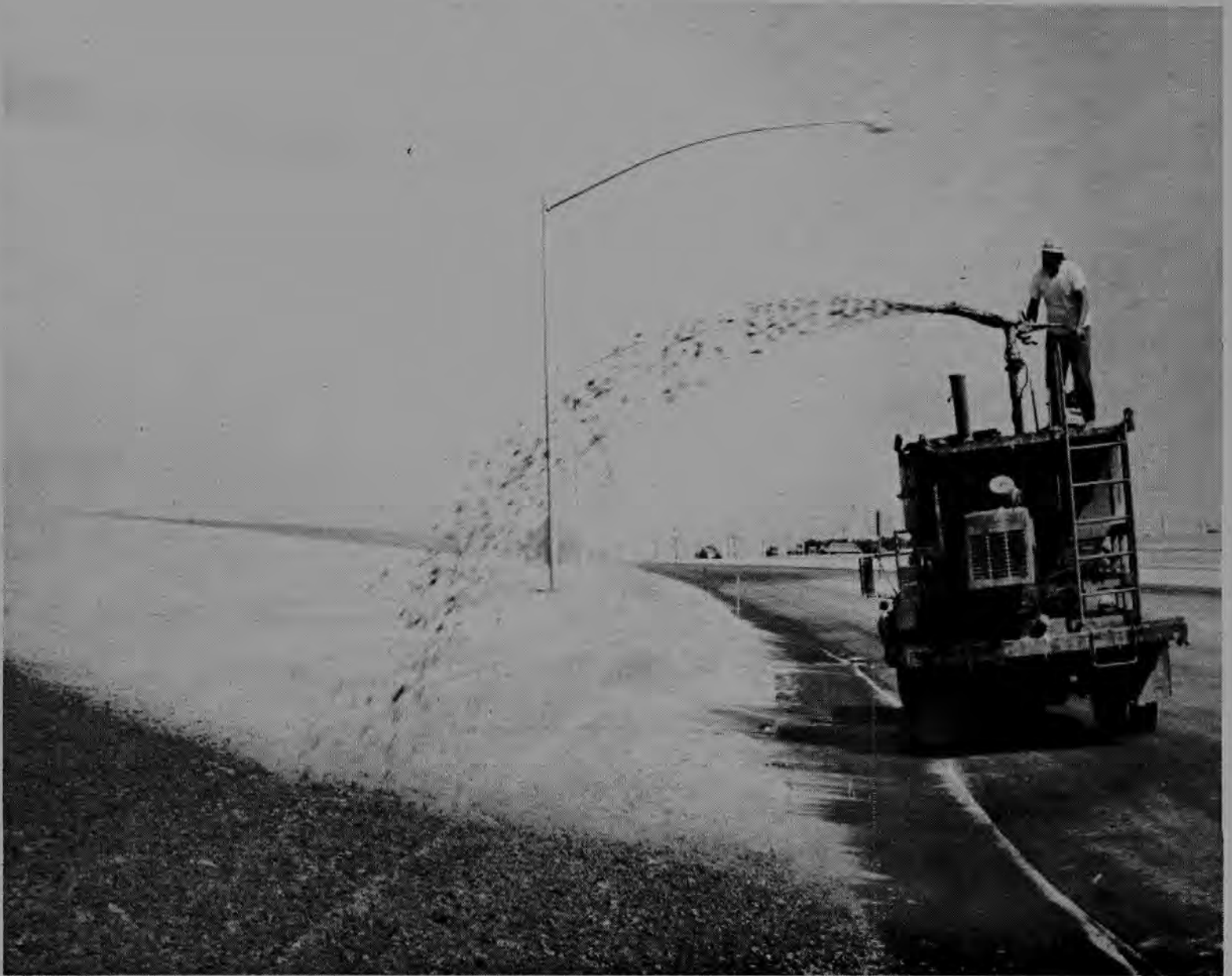
INSTANT LANDSCAPING —The new method of landscaping on Freeways is done by spraying the seeds mixed with a mulch under pres-
