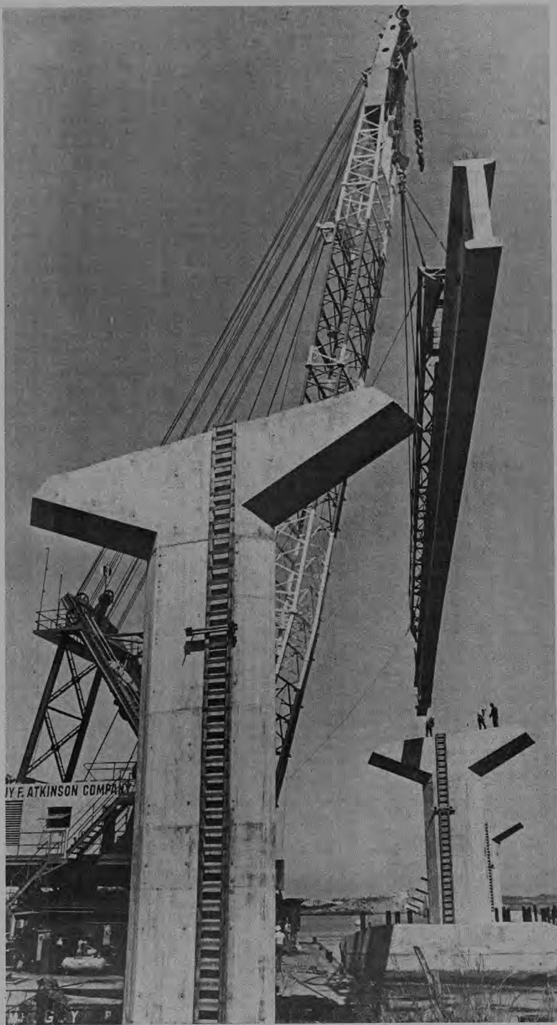
HIGHEST AND WIDEST span of the Eureka-Samoa bay bridge gets the first of four girders, as three workmen atop the far pair are dwarfed by the giant crane and structures. The first two barge loads of the specially fabricated girders arrived from Tacoma, with another due soon. The rest of the 164 required will arrive by the last of October. The $5.25 million State Division of Highways is expected to open to traffic in mid-1971.
