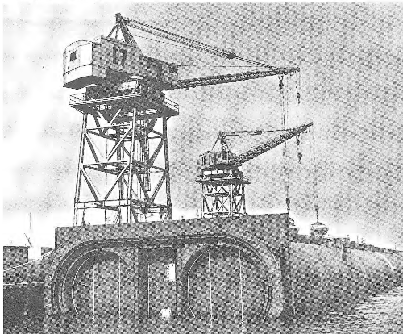
PLACING CONCRETE in floating tube section with 100-foot-high rail mounted cranes and 5½-yard buckets.
