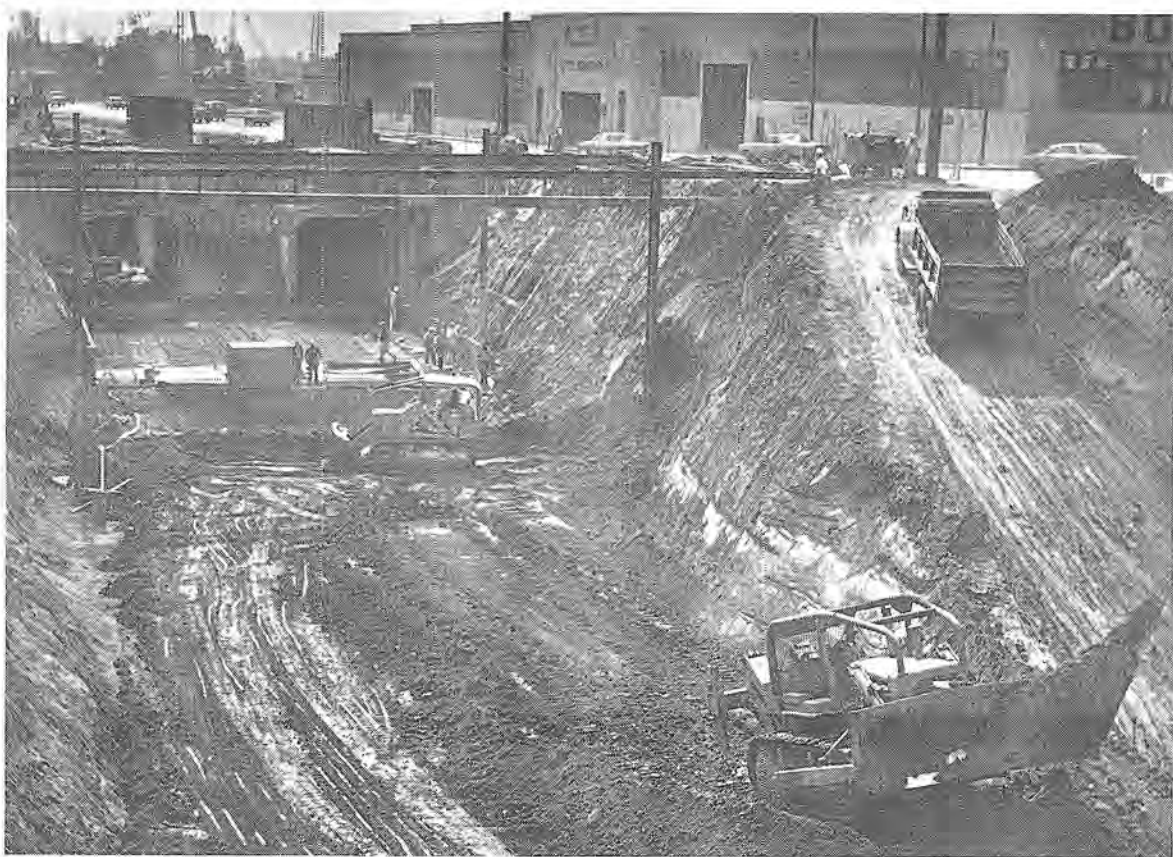
TRAIN PATH —Twin Bay Area Rapid Transit subway tunnels are clearly evident at 9th and Oak streets in Oakland. The big ditch in the foreground is the excavation for the Lake Merritt subway station. The squarish-appearing tunnel will be
