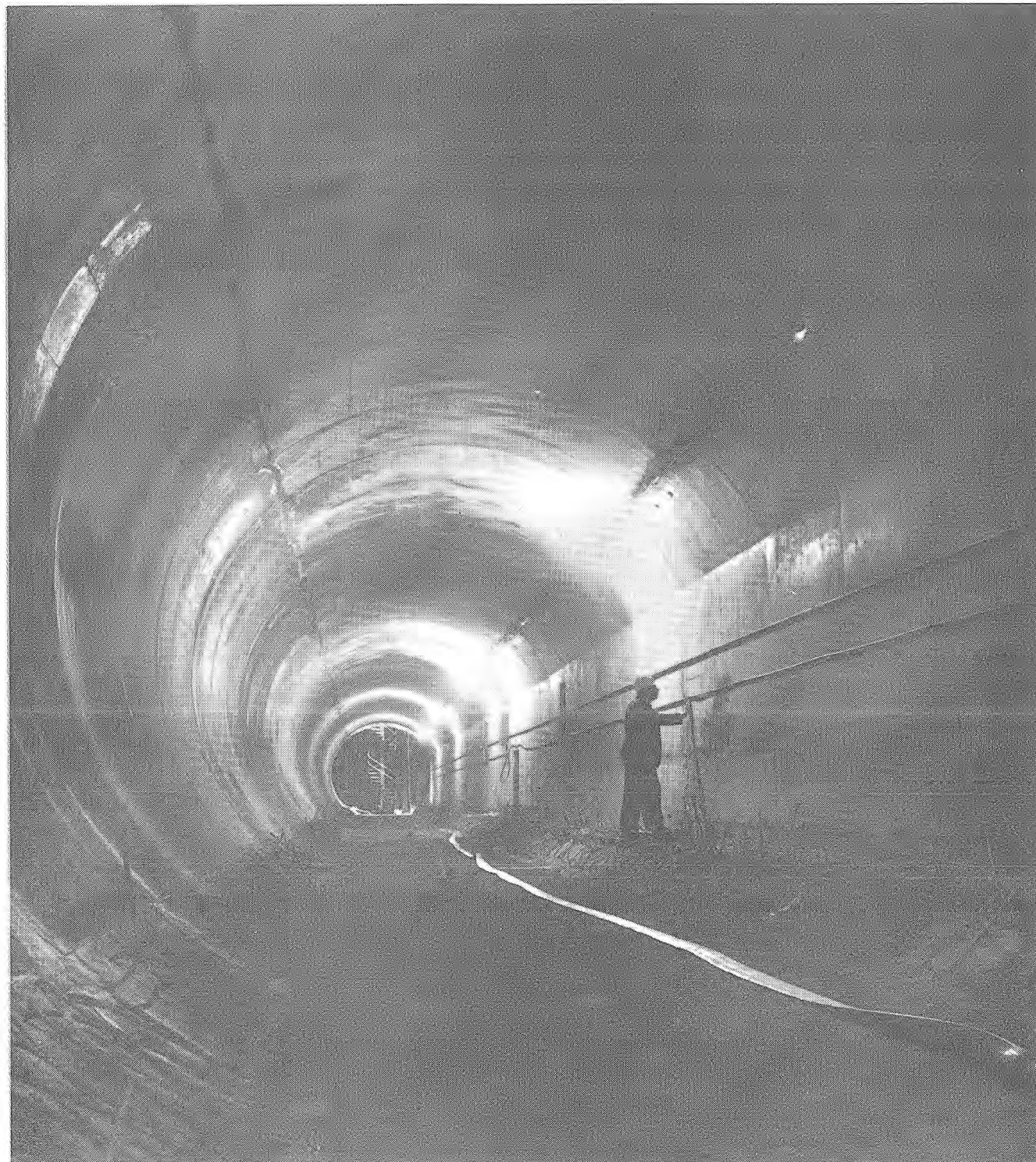
FIRST VIEW inside tube of the first section of the underwater Trans-Bay Rapid Transit Tube which will extend along the floor of the bay between San Francisco and Oakland. Two of the 57 massive steel and concrete sections that will comprise the four-mile tube—longest
