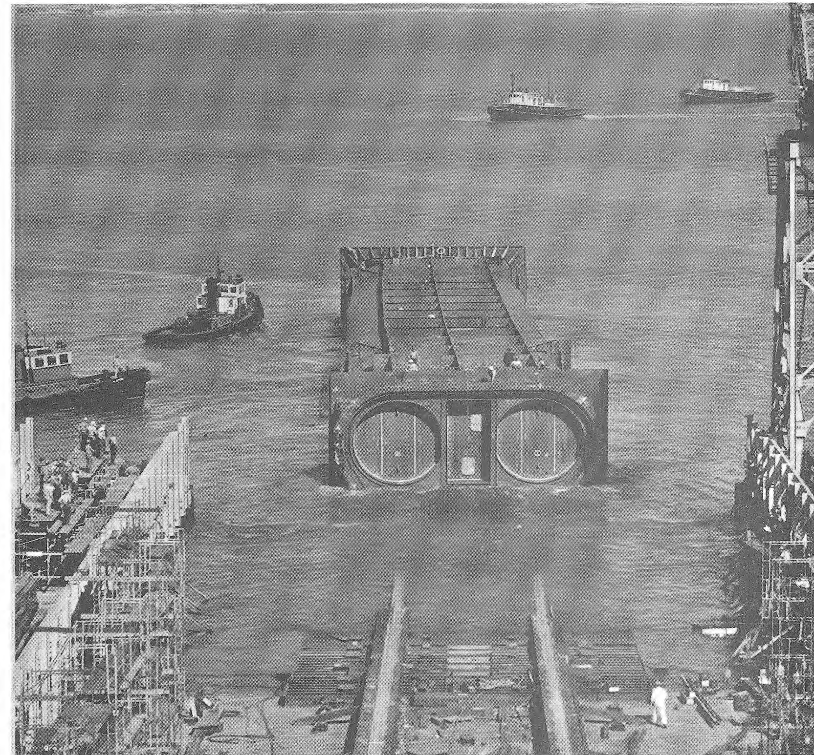
LAUNCHING FIRST section of the Trans-Bay Tube. The steel sections—averaging 330 feet in length—are fabricated on shipways, launched and floated to an outfitting dock where concrete interiors
