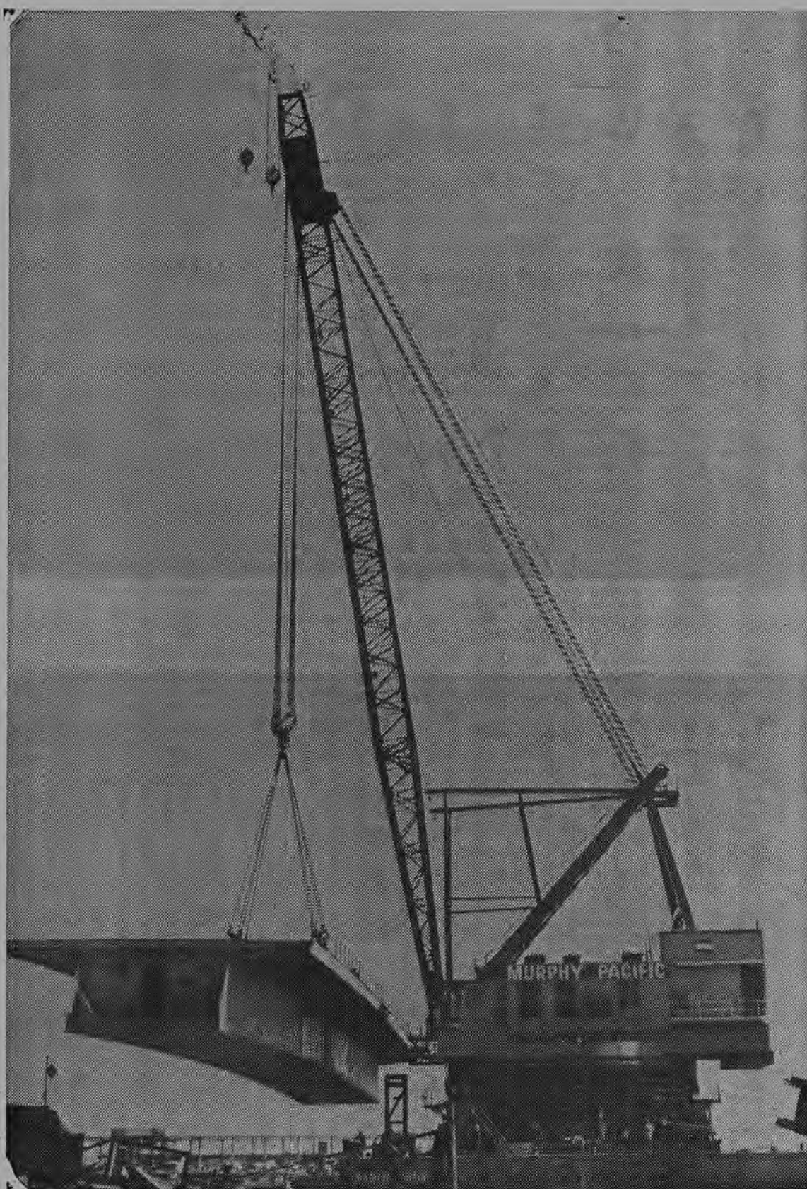
BIG PICKUP —Lift for the 300 ton section of the Sacramento River Bridge job is shown in process above. Operator is Brother John A. Paro, Brother Joseph "Joe" C. McCarthy is the Deck Engineer and Brother Leslie M. Mears is the Oiler.
