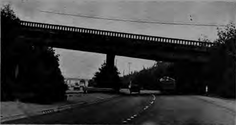
THE OLD . . . The Arcata 11th Street crossing represents an earlier solid style of spanning roadways, which is some 15 years old. Notice the heavy pillar in the center, which blocks a drivers view and presents a potential collision object. —Times-Standard photo.
