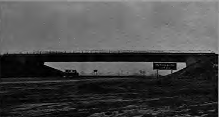
THE NEW . . . The longest span possible for this type of overpass is this 180-foot crossing which spans U.S. 101 North of Arcata. The crossing cuts the accident rate from six to one accidents per year.—Times-Standard photo.
