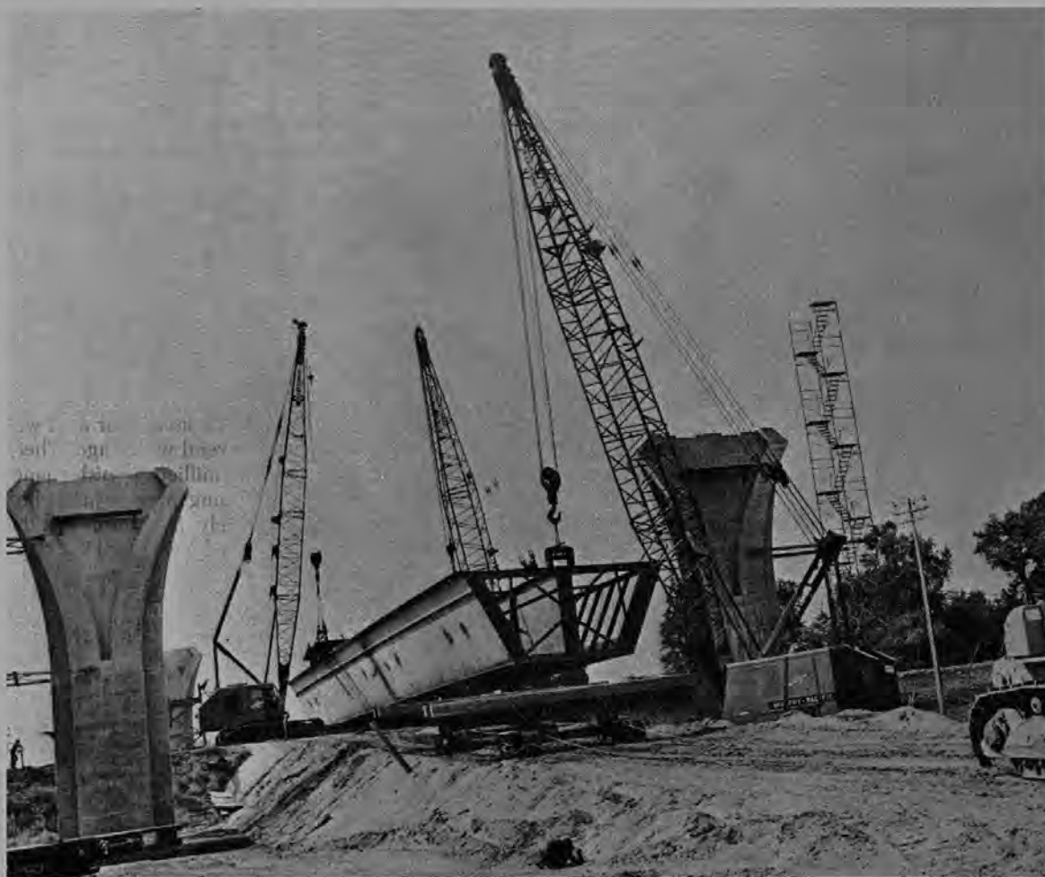
BIG LIFT as Murphy Pacific calls on three cranes to set in place one of the huge girders being used on the Interstate 880 highway job. This one weighed two hundred and sixty-five tons and crane
