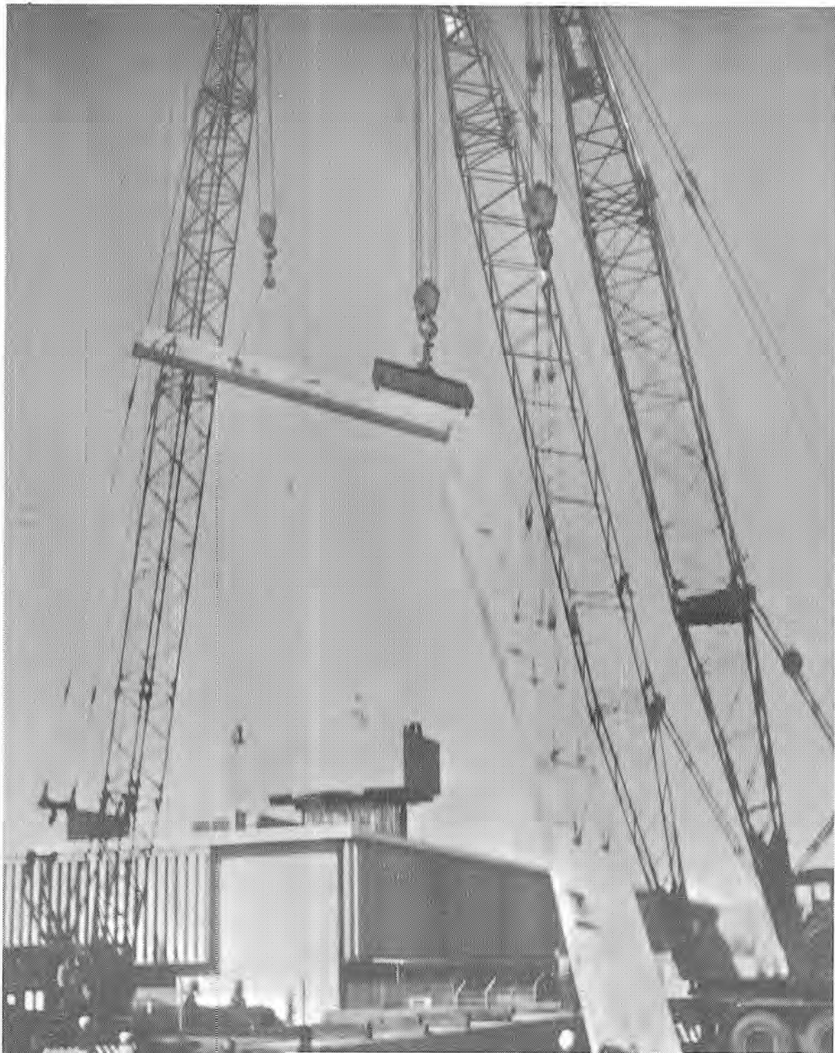
TOUGH TRIO of cranes manned the frontline in the nearly completed job on the new Philco plant in San Jose. Job consisted of erecting two 40-ton concrete columns and twelve 63-ton L-shaped concrete bents. Three cranes, 140-ton, 100-ton and a 60-ton were needed for the job.
