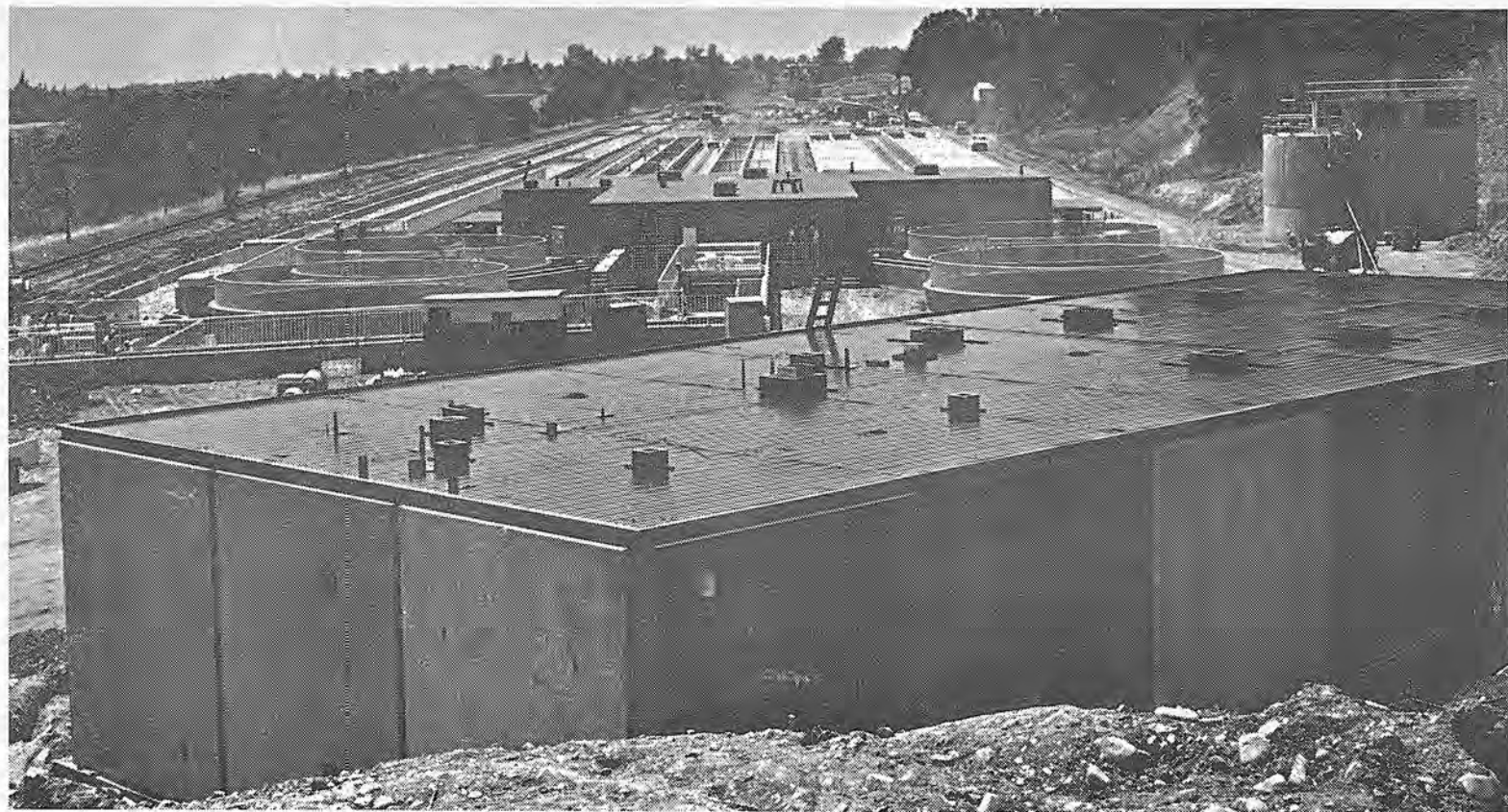
HATCHERY PANORAMA —Construction of the $3 million Feather River Hatchery was completed in time for the fall run of salmon and steelhead. Building in foreground is the hatchery's administration and warehouse facility. Beyond the structure are the four circular "holding tanks" where the fish will be held after sorting until they are ready for natural or artificial spawning. Beyond the tanks is the fish handling building, where the salmon will be sorted, some stripped of their eggs for artificial incubation, others marked
