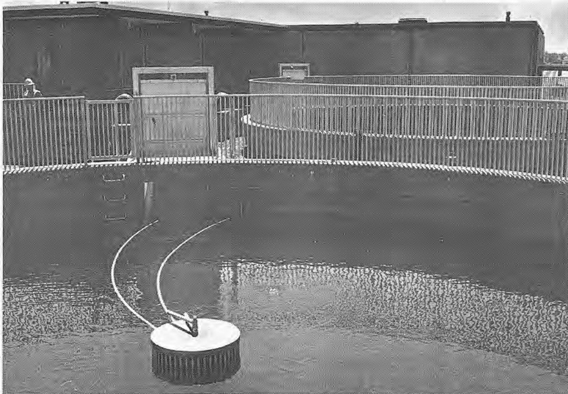
HOLDING TANK —Salmon and steelhead will stay in four holding tanks similar to this one until they are ready to spawn. When ready, the fish will swim through gated channel at far side of tank
