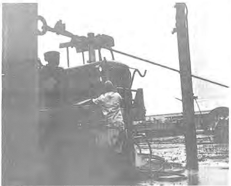
Workers performing gunking of machinery were subject to being pushed into pond by pressure. Wire fence stops such occurrences.
