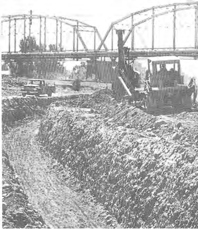
Power shovel and Cat excavate path of the 2,000-foot fish ladder. Officials say 16 million fish will be hatched annually at this site.
