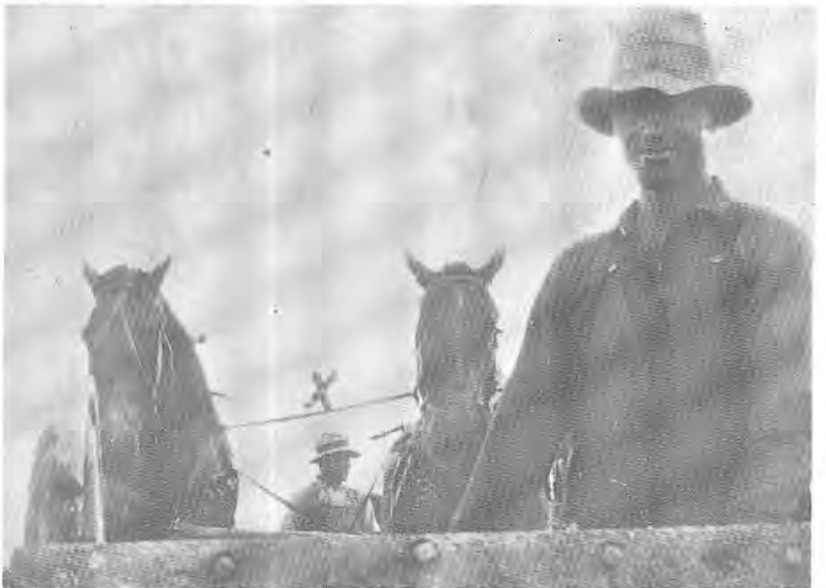
First so-called "bulldozer" in Canada was more of a "Muledozer." A slab was pulled by the mule and when it was loaded, the operator lifted it and dumped the load. Crews built roads, not highways.
