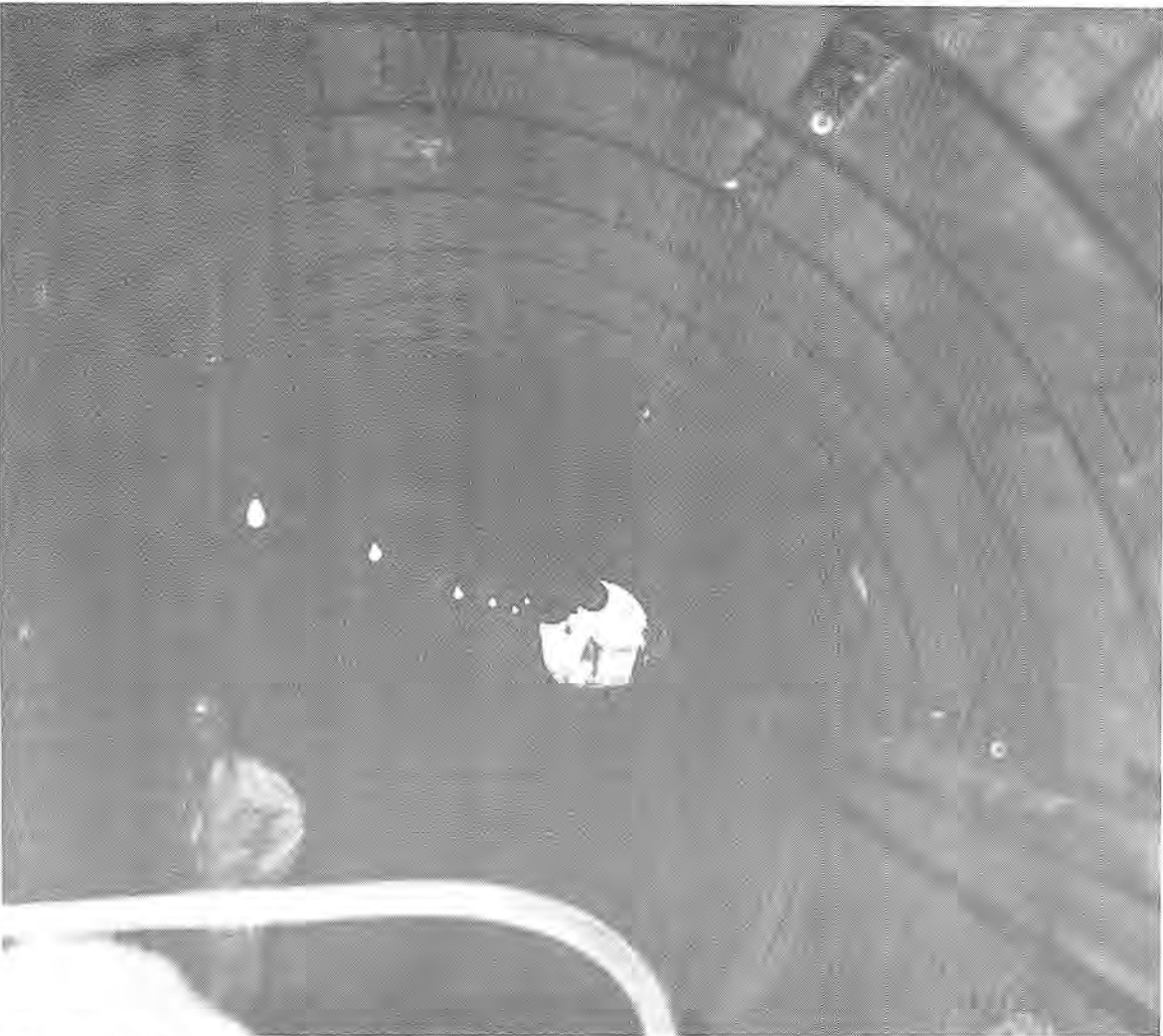
North segment of the Crystal Springs Bypass tunnel is progressing smoothly. Alignment is being controlled by means of a laser beam. The two segments will be joined late this year or early 1968.
