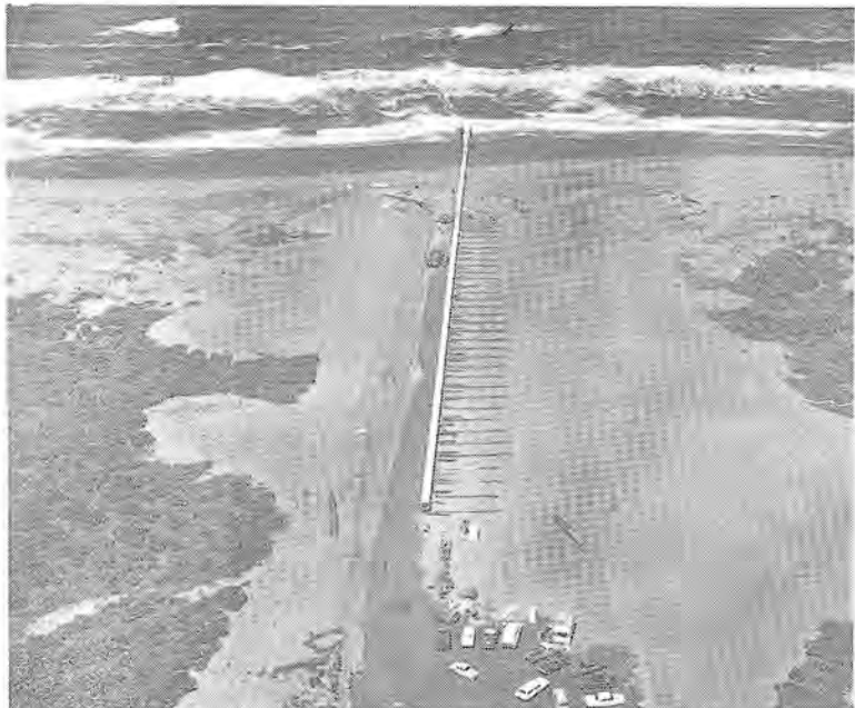
New pipeline being constructed near Samoa for water outlet for pulp mill will be completely built and pulled to sea where it will be laid.
