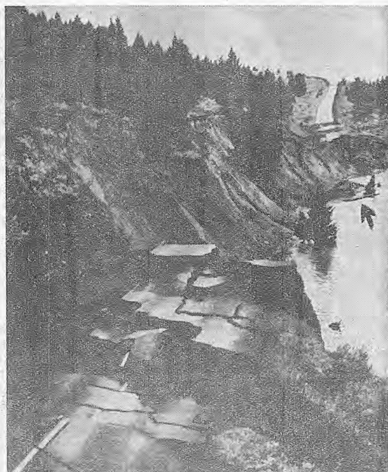
BROKEN ROAD to disaster. When the Montana earthquake struck, this hillside slid into Hebgen Lake, carrying several hundred feet of Highway 1 and a cabin with it, the worst of four areas. Arrow points to submerged cabin. Heavy equipment was moved quickly into the quake area.
