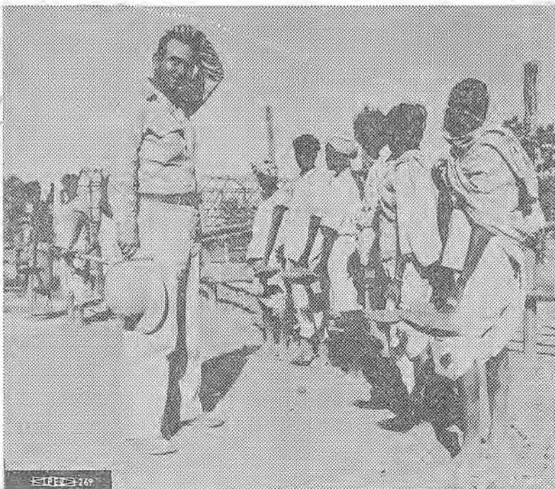
Brother Ted Bankston, with the U. S. Army "somewhere in Burma," is shown with his "gang" of coolies, who are building a road by hand. Carpenters on this job get $3.20 a week, and laborers get $1.20 a week—big wages for that country!
