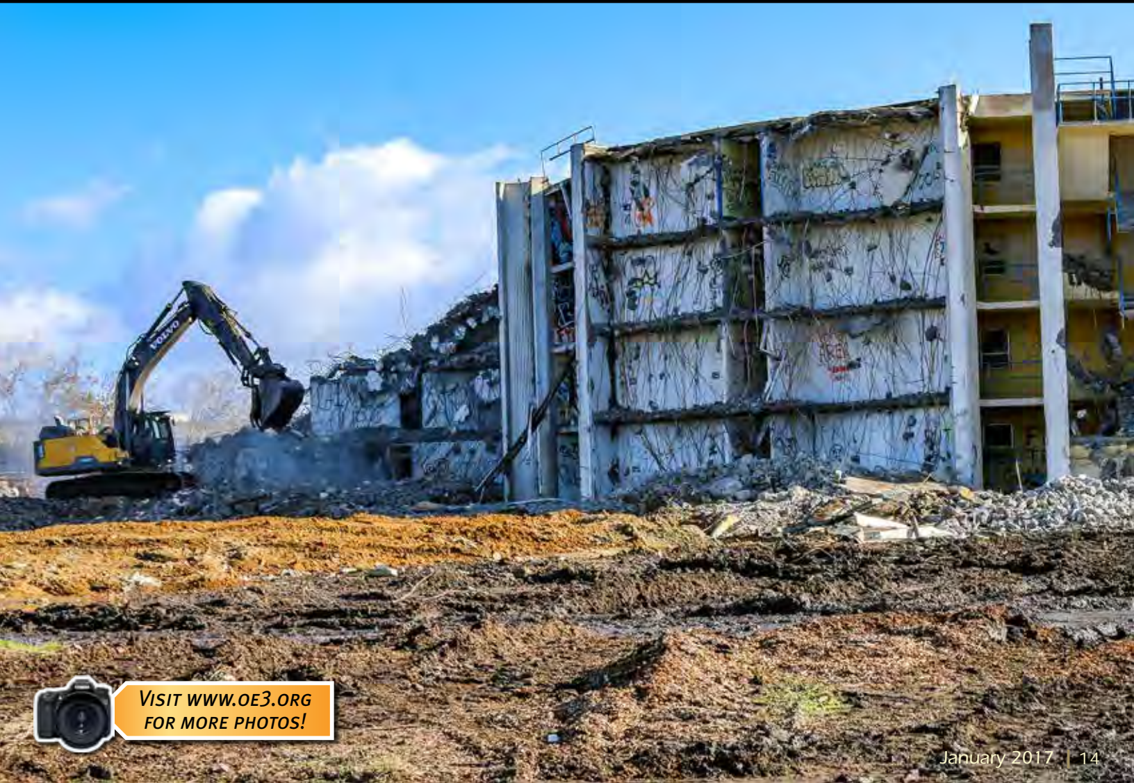
Above: Excavator Operator Jose Lugo separates the rebar into neat piles for Rock Truck Operator Ricardo Aguilar, while Ampco North Excavator Operator Jose Parra demos the old Star Barracks on Treasure Island, below.
