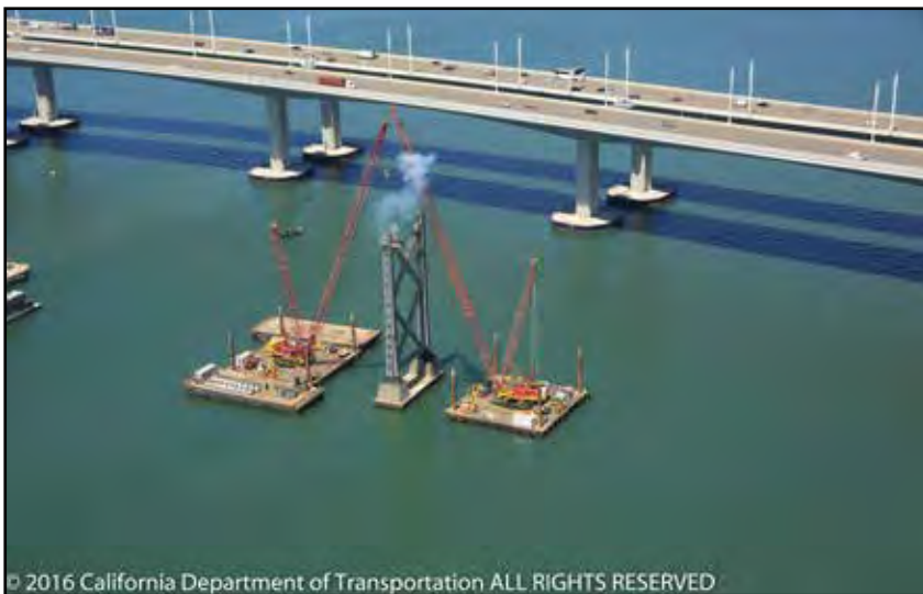
The implosion of the few remaining piers takes place as part of the old Bay Bridge demo.
