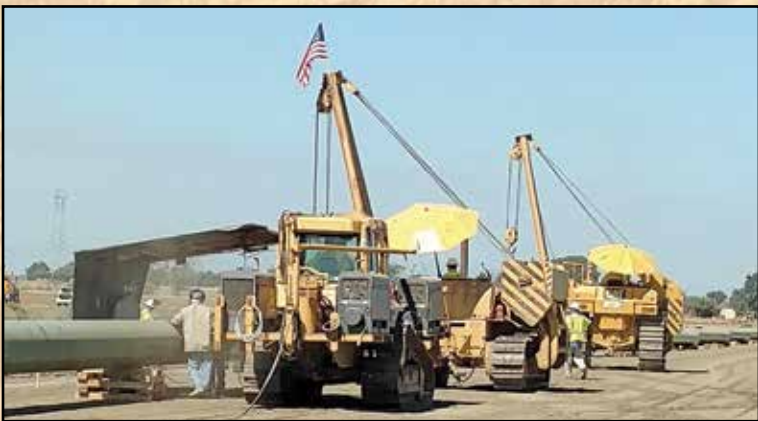
Members with Abercrombie Pipeline Services, Inc. operate side booms in Woodland.
