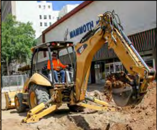
Bill Nelson Construction Operator Esequil Barragan works on storm drains as part of the Fulton Mall revitalization.
