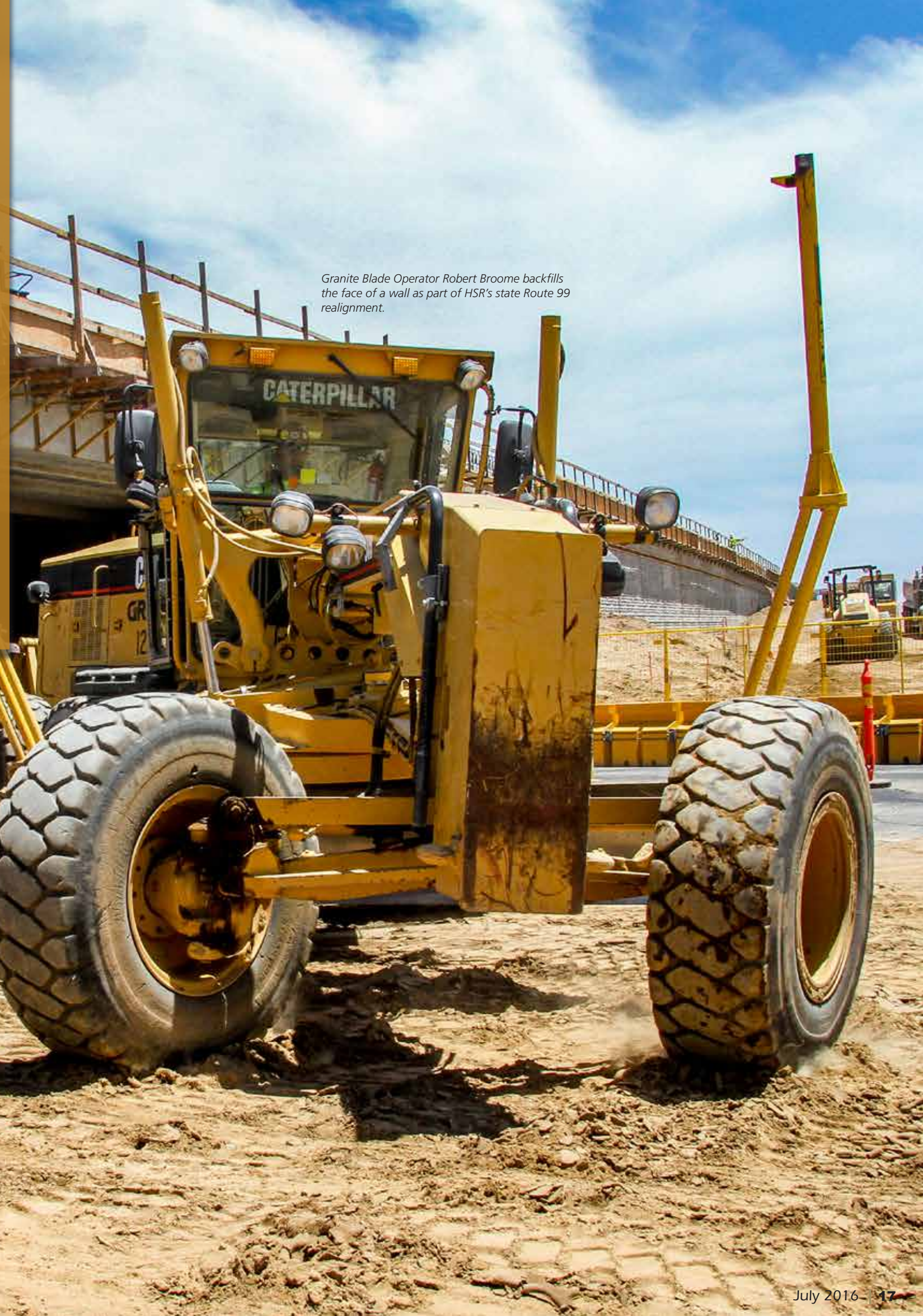
Granite Blade Operator Robert Broome backfills the face of a wall as part of HSR's state Route 99 realignment.
