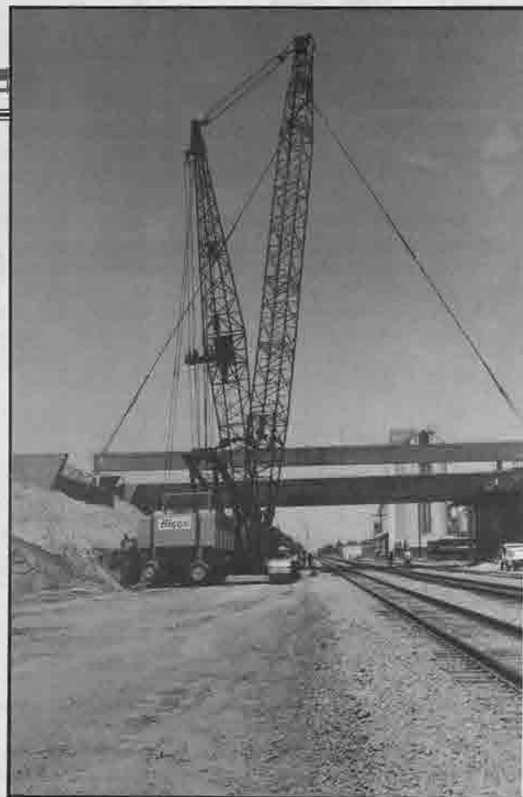
Right: Biggie Crane and Rigging recently moved in one of the largest cranes ever used in the Fresno area to move 19 bridge beams for the Hwy. 180 "Gap" freeway project. The crane was an American 1125 with a 600-ton lifting capacity. The Skyhorse on the rear of the crane weighed 200 tons. The 19 beams, which took three days to move into place, weighed 238,000 pounds each and measured 134 feet in length. Above: the crew was from left oiler Jay Brown, operator Randy Burke and mechanic Ken Bacon.
