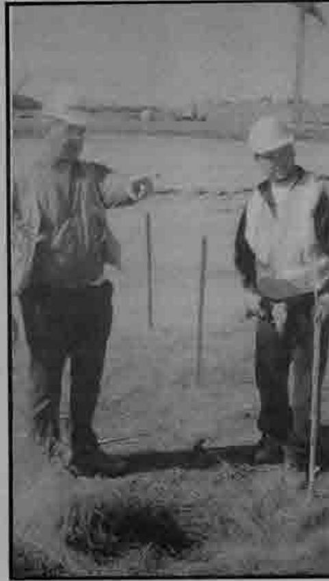
Below right: Gradechecking instructor Jack Kraft, left, shows third-period apprentice Joe Villarreal how to mark the stakes for a slope.
