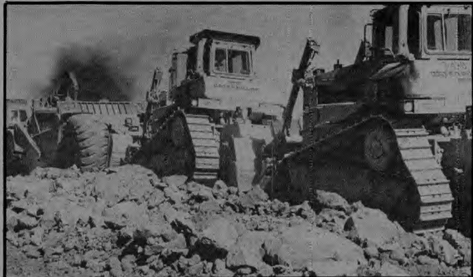
Cat D-8L operators working for Granite Construction team up to push scraper operator Mike Souza through an extremely rocky stretch of the Hwy. 65 Roseville Bypass (above). To the left is the causeway which comprises part of phase 1 of the project. MCM is the general contractor on this section with Teichert subbing about $5 million of the work. Mechanic Jacquie Bowerman and dozer operator Bob Harris (below) take a lunch break on Granite's job.
