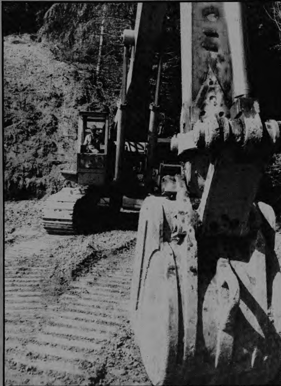
Cecil Martin mans backhoe (above) while Harold Grant handles dozer.
