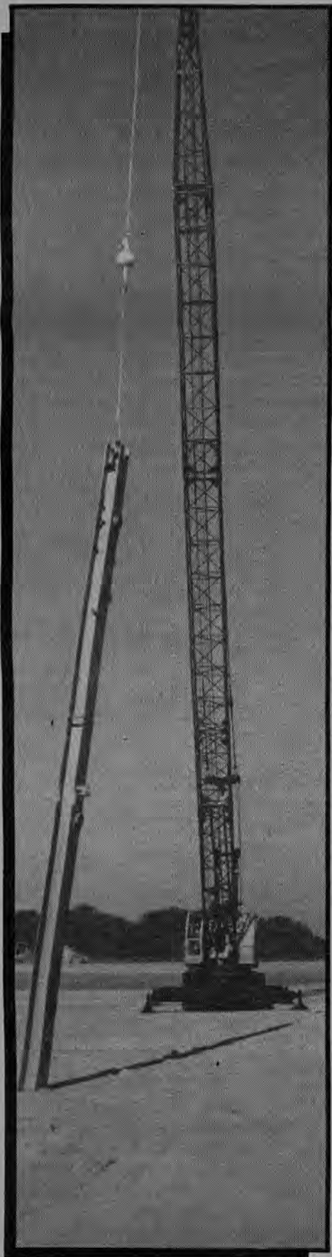
Apprentice practices lifting beam.
