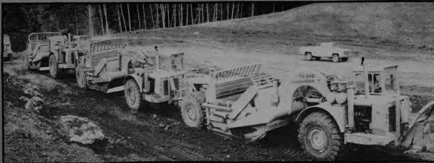
Three cans line up in a push-pull operation on the northern spread of the project.
