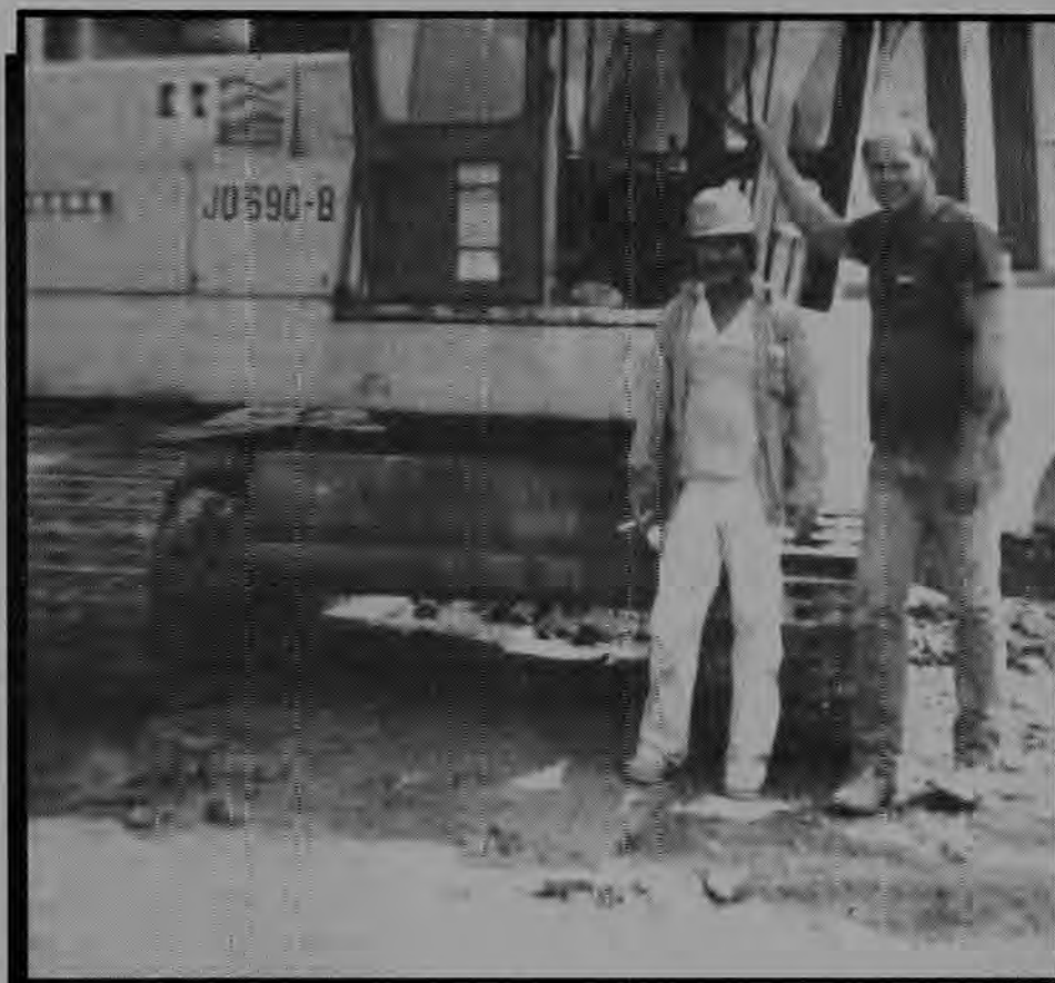
Pictured above are oiler Justo Daoang and backhoe operator Richard Robb. They are working for R & R Construction on the Kapiolani Community College project.
