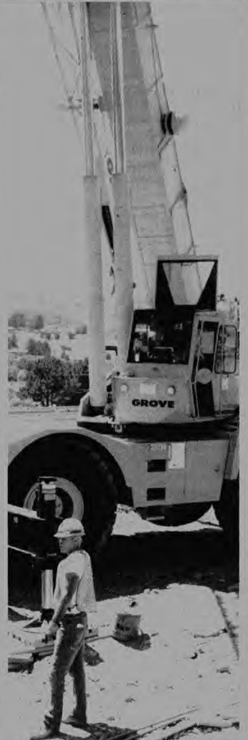
Setting foundation forms on the San Pedro Rd. overcrossing is operator Jim Scagliola and oiler Norm Sweet.
