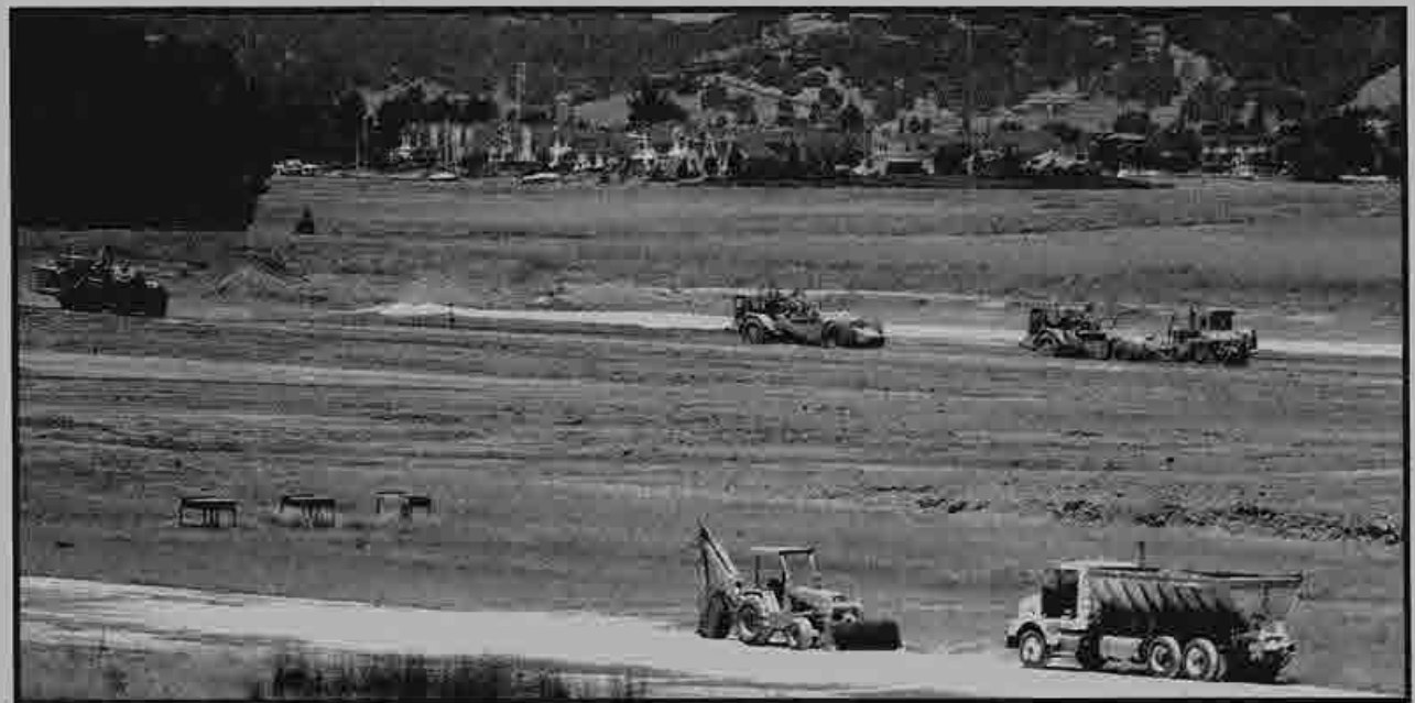
Left: Mechanics Stan Olsen, left, and Dave Schmidhans keep the iron moving. Below: Scrapers work on the wetlands restoration section of the projects, which consists of 33 acres that will replace wetlands lost with reconstruction of the landfill.
