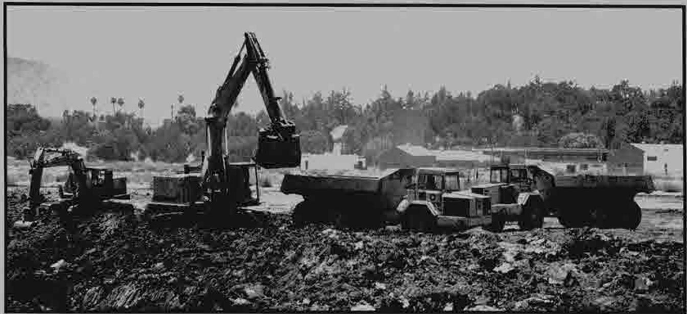
Top: Excavators dig up top soil used to put over the landfill's clay cap.
