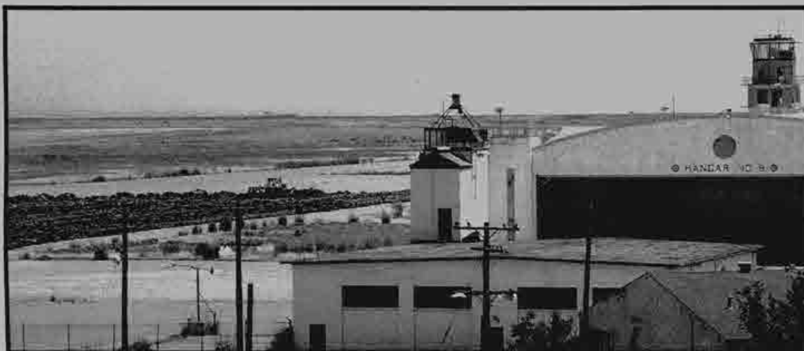
Left: a lone compactor, center and slightly to the left, disks drying clay that was spread out over parts of the base's old runway and taxiway so it could be conditioned and dried to a moisture content of 22 percent. After that, the material was transported back to the landfill area and used to line and cap the old dump. Where hangar No. 9 now stands will lie portions of a business and industrial park being developed by the New Hamilton Partnership.
