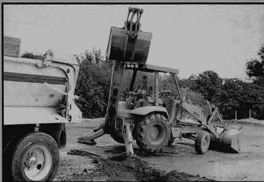
An operator digs a drainage trench on the Occidental Road project in Santa Rosa, where North Bay is widening and rehabilitating about 1.5 miles of this vital thoroughfare.
