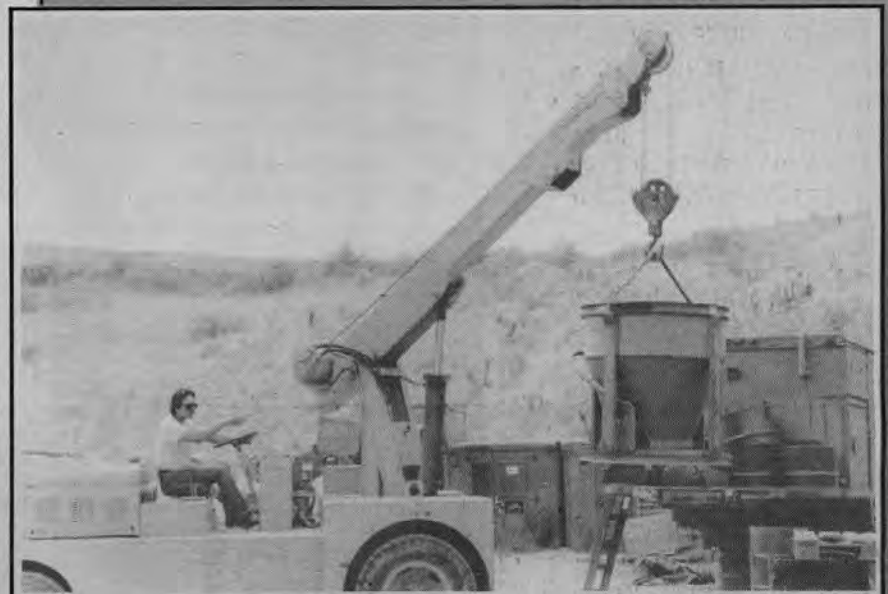
Pictured left is 25-ton P&H crane at training site. Each class member practiced signaling to the crane operator to land a load in blind. Pictured above is Nyle Boyce, Shawn Craig and Tom Nimrod. Below, Tom Nimrod practices picking up and placing load.
