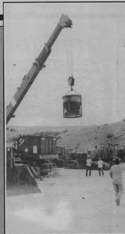
Pictured left is 25-ton P&H crane at training site. Each class member practiced signaling to the crane operator to land a load in blind. Pictured above is Nyle Boyce, Shawn Craig and Tom Nimrod. Below, Tom Nimrod practices picking up and placing load.
