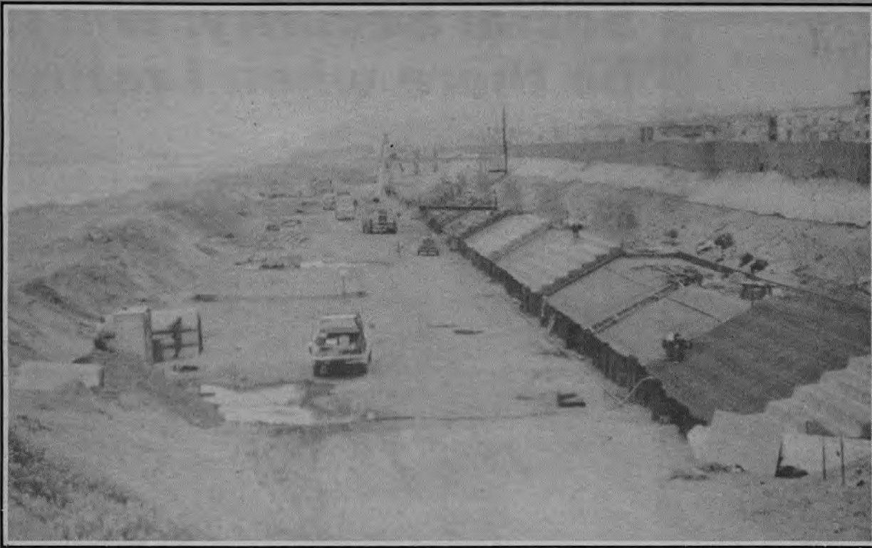
Local 3 members build massive sea wall at San Francisco's Ocean Beach.
