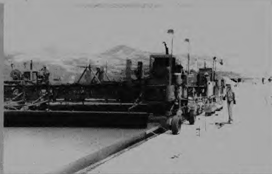
Local 3 members Cheryl Osborn and Leisa Abott inspect the finish concrete laid by the Gomaco 5000 concrete paver.
