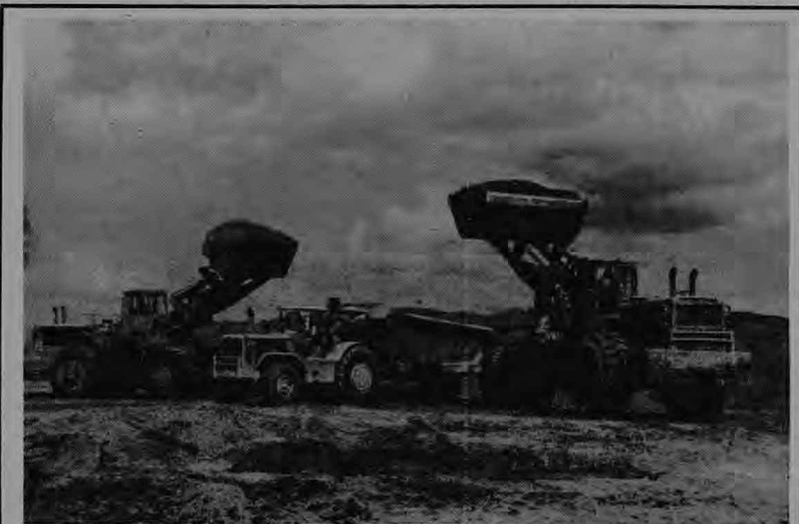
Operating Cat 992 loaders, Local 3 members working on the $8 million I-80 bypass at Battle Mountain load borrow material into tandem bellydumps.
